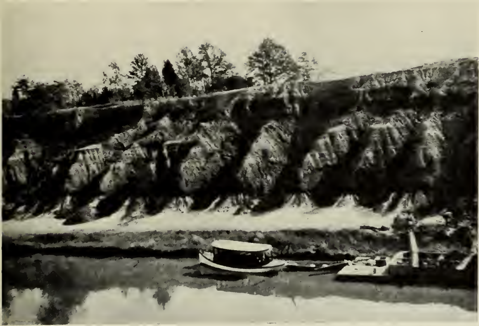
FIG. 1.—VIEW OF SECTION ALONG CHESAPEAKE AND DELAWARE CANAL, SHOWING MATAWAN FORMATION OVERLYING MAGOTHY FORMATION.
