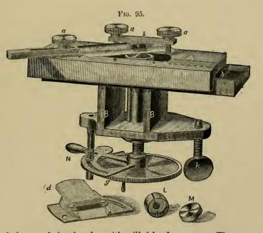
steel clamp and shoe b and c, with milled-head screws a. The carriage runs on a solid iron track h and B, which is held to a table by clamp screw k.
