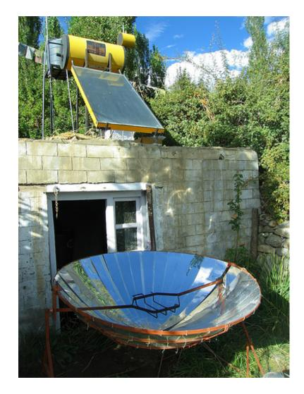
Figure 4.12: A solar cooker and a solar water heater in India. The solar water heater is on the roof of the building. The solar cooker is the silver dish in front of the building.
