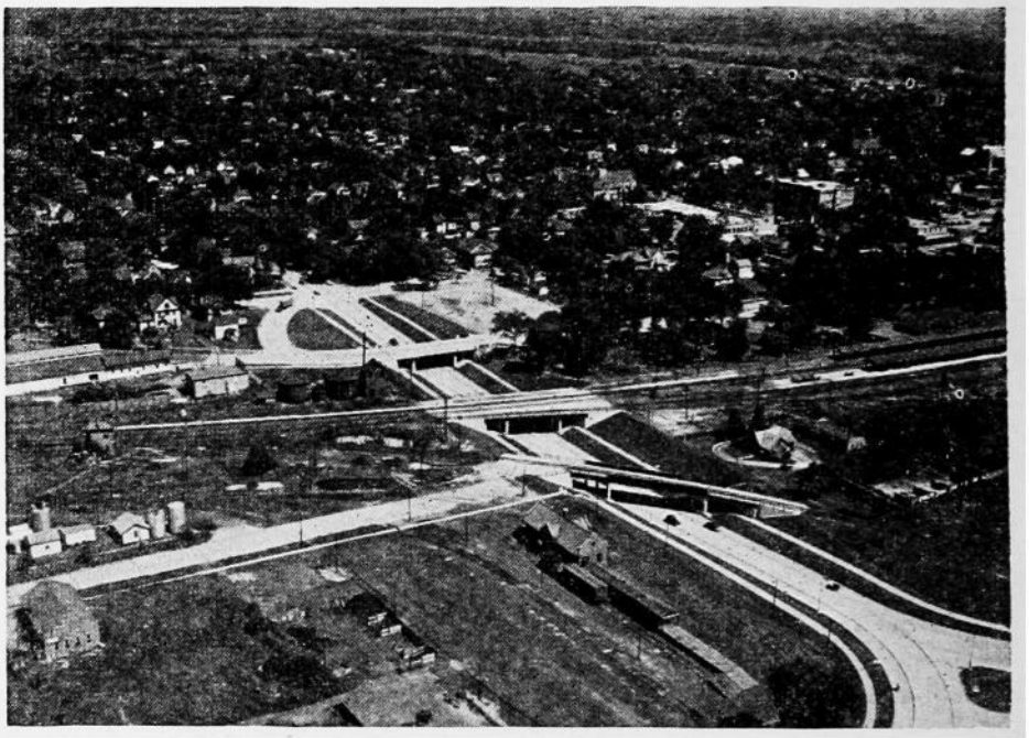
Subway and Traffic Separation Project at Ames
