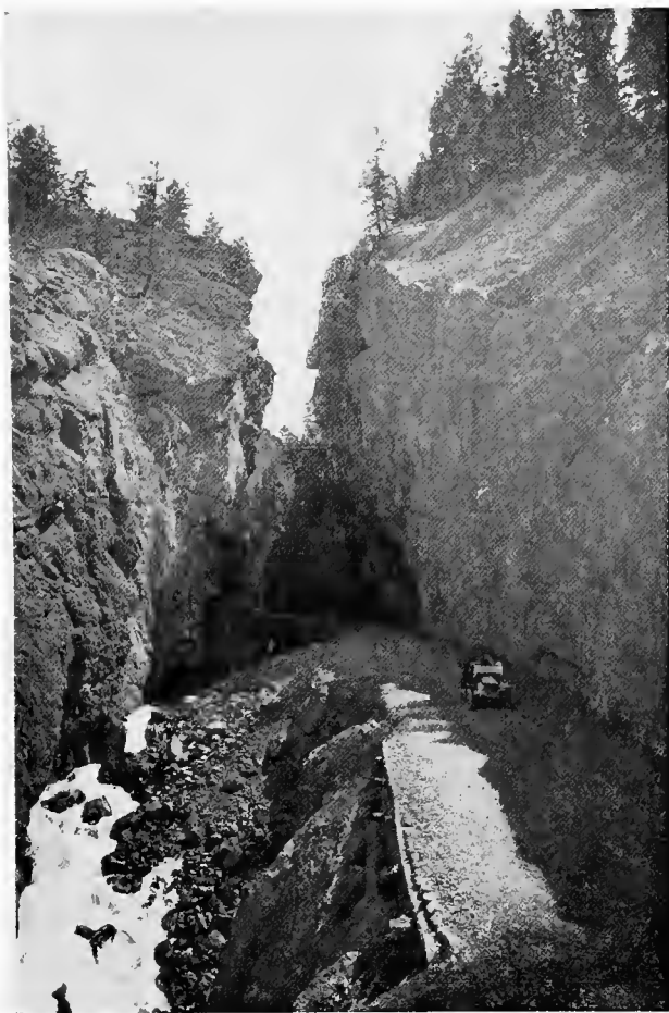
IN SINCLAIR CANYON, ON THE NEW HIGHWAY FROM THE COLUMBIA RIVER VALLEY, TO BANFF, ACROSS THE ROCKIES
