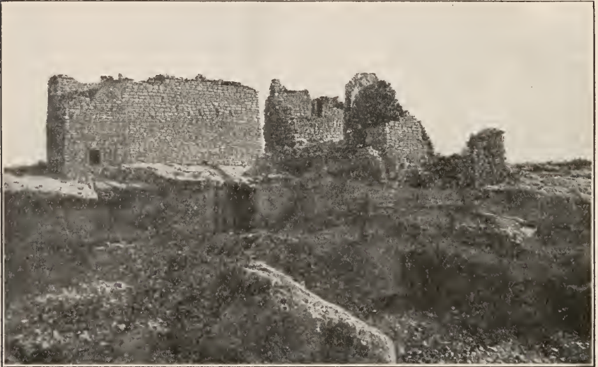
Fig. 3. Tower ruin in Ruin Canyon, Utah.
