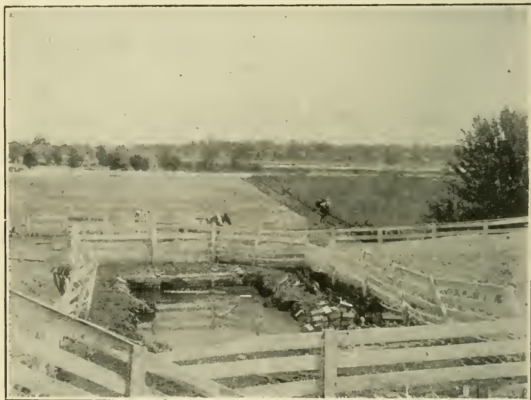
Old Cesspool, showing method of disposal of sewage prior to new system.
