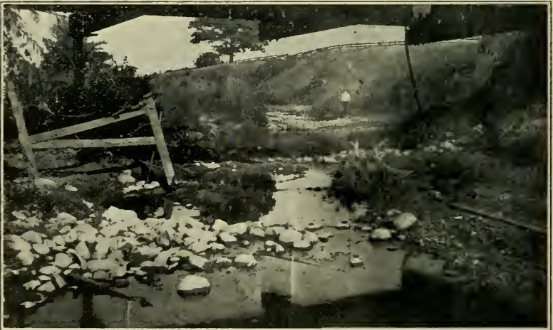
Fig. 7. View up the channel of the outlet at the greater dam. The depth of the valley is shown by the altitude of the right abutment in the background. The evidence of the ascending erosion line is in the foreground.
