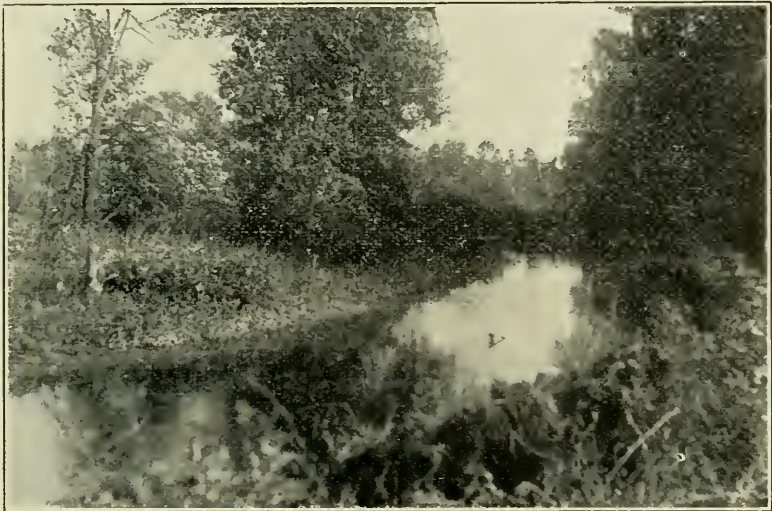
Fig. 5. View of the channel and abutments of the upper or lesser dam. From the condition of the vegetation in the foreground, it is evident that the stream's gradient is small. Upon the left and right the surface rises abruptly to 12 feet, and is covered with heavy mesophytic trees. The soil is sandy. This is a place where vegetation is capable of closing the drainage lines.
