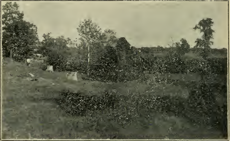
Fig. 6. View across the valley from the left abutment of the lower or greater dam. The width of the valley is here about 165 feet, with the earth walls rising abruptly 22 feet on either side. The soil is a glacial deposit, sand predominating.
