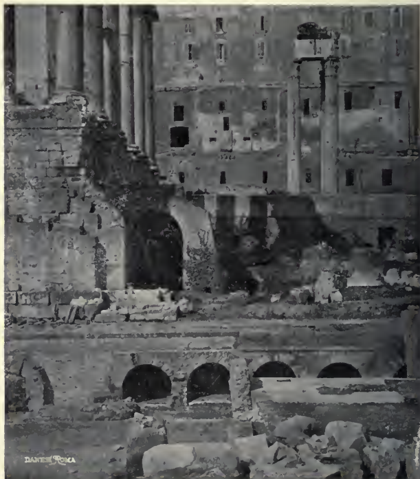
Fig. 24. Substructures of the Clivus Capitolinus. (in the background the temples of Saturn and Vespasian).
