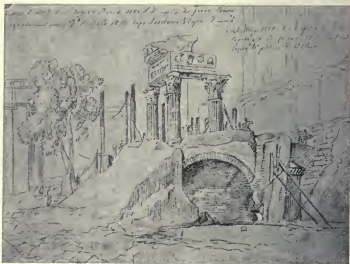
Fig. 41. Excavation near the temple of Vespasian in 1812.
