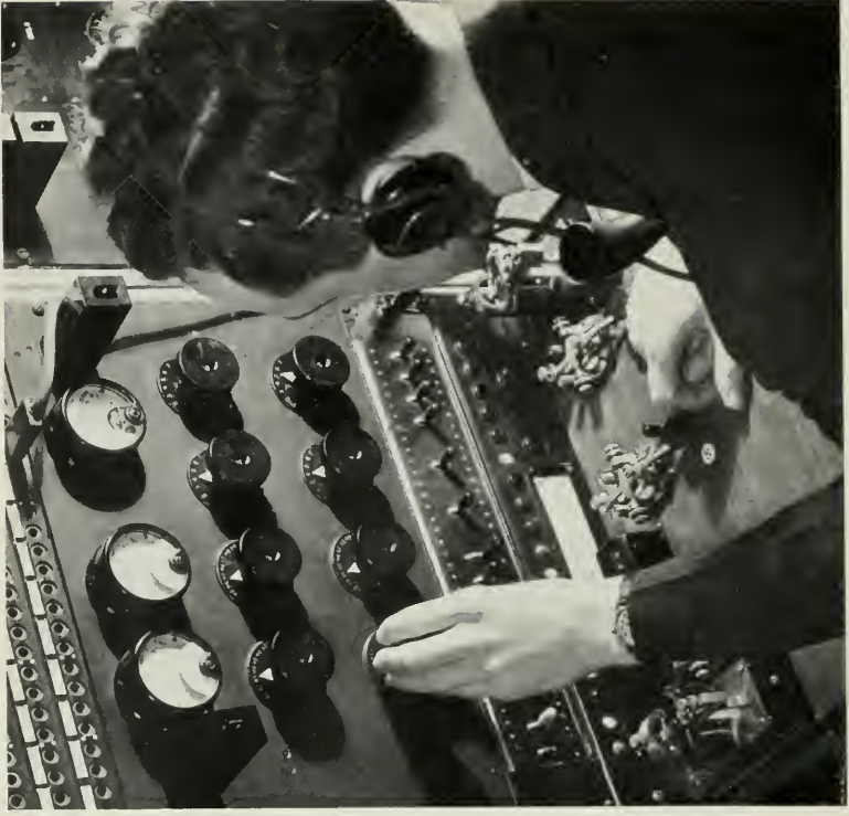
A CIRCUIT PATROLMAN ADJUSTS RADIO TELEPHONE CIRCUITS.
