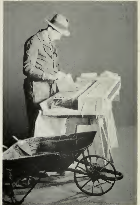
FIG. 10. WORK BENCH AND TRAYS DESIGNED TO FACILITATE THE MAKING OF MORTAR BANDAGE JOINTS.
