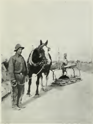
Stone-Boat for Stringing Wires
