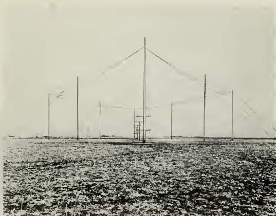
FIG. 6. HORIZONTAL DIAMOND TYPE ANTENNA CONNECTED FOR TRANSMITTING.
