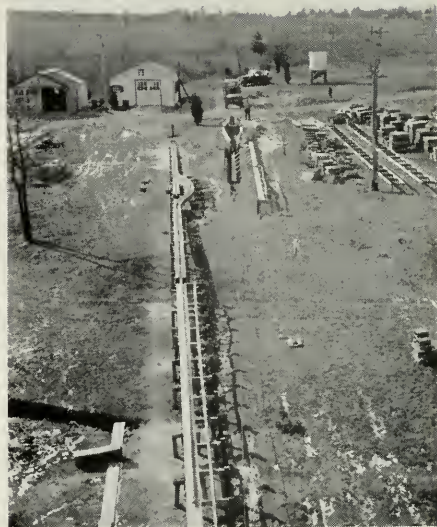
FIG. 2. PARTIAL VIEW OF FIELD LABORATORY AT CHESTER, NEW JERSEY.
