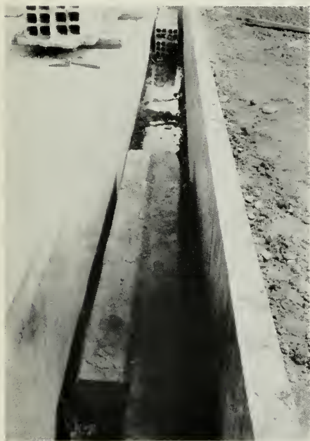
FIG. 3. VIEW OF ONE OF THE FLOODING TRENCHES AFTER A TEST.
