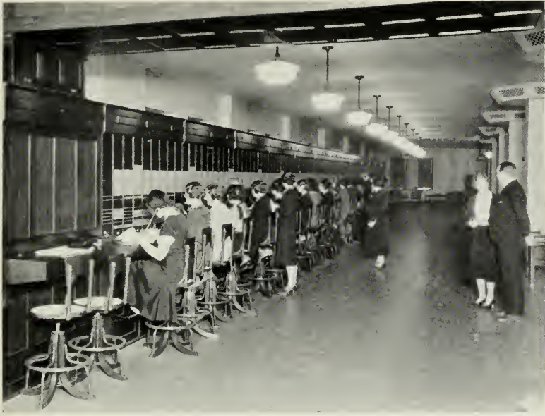
FIGURE 1. MANUAL SWITCHBOARD USED IN CONJUNCTION WITH DIAL EQUIPMENT.
