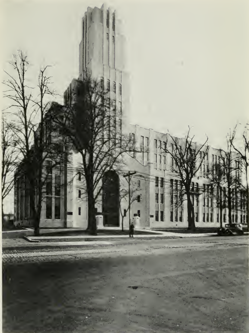
WESTERN ELECTRIC CO. DISTRIBUTING HOUSE, BOSTON, MASS.
