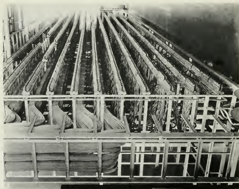
FIGURE 3. DISTRIBUTING FRAME.
