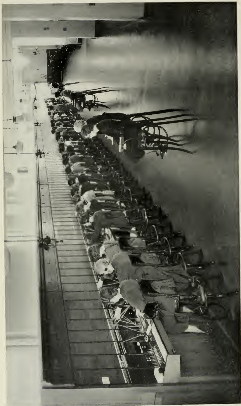
LATEST TYPE DIAL "A" BOARD FOR HANDLING CALLS IN A DIAL OFFICE THAT REQUIRE THE SERVICE OF AN OPERATOR. (See page 38.)
