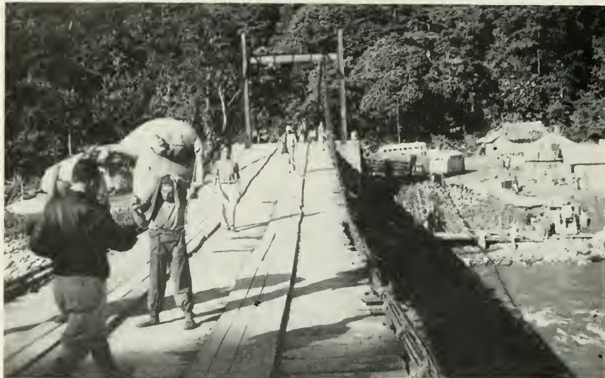
1. Transshipping cargo by hand across the Humadea River on the frail suspension bridge.
