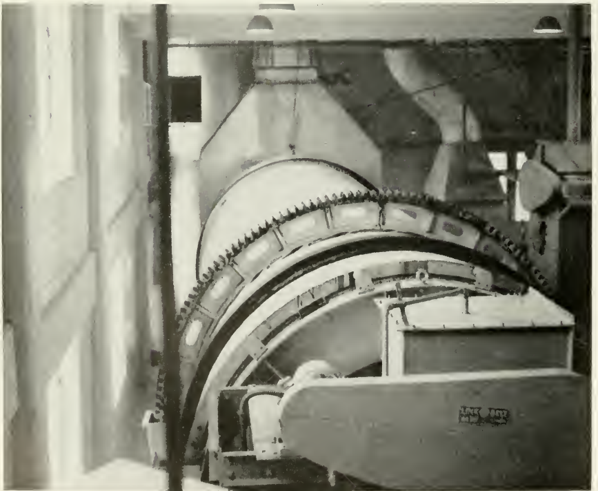
2. Rotary sludge dryer, Fairfax County sewage-treatment works, Va.
