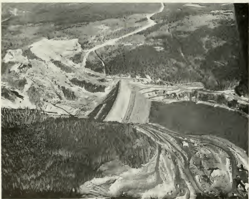
2. Nechako aerial view of dam area.
