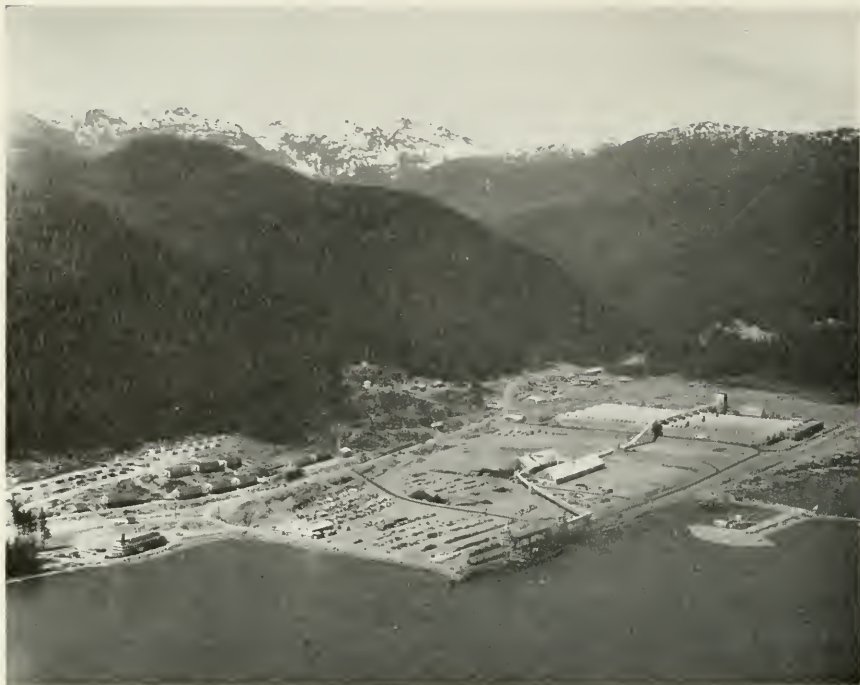
1. Aerial view of dock and smelter, Kitimat, British Columbia. Delta King , former Sacramento River stern wheeler, is at left, now used as a workers' dormitory. Her boilers also furnish steam to heat hospital and other buildings.
