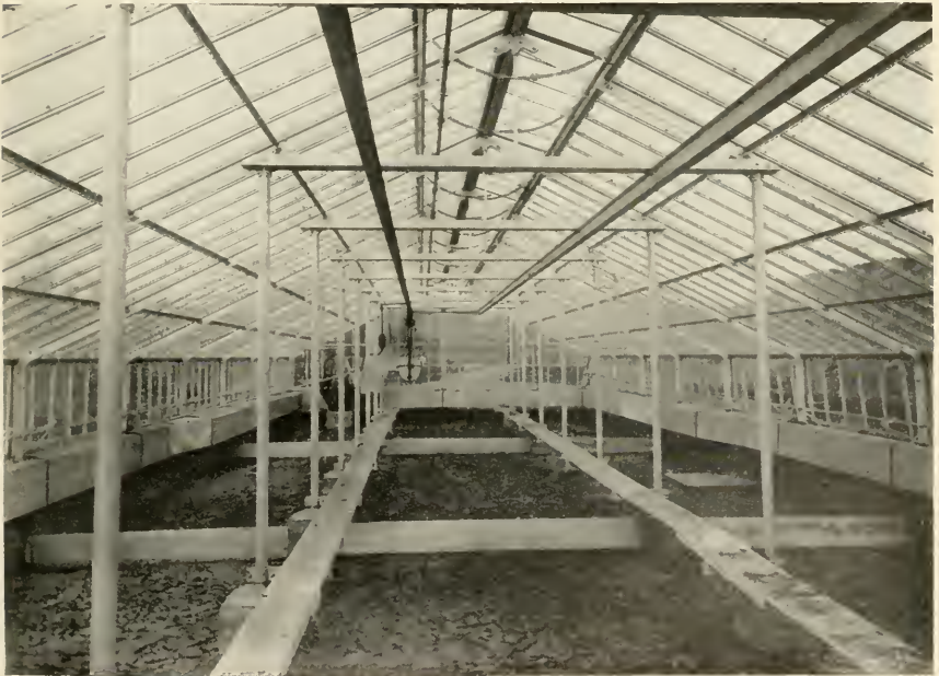
2. Covered sludge-drying beds, New Lexington, Ohio. (Lord & Burnham Co.)
