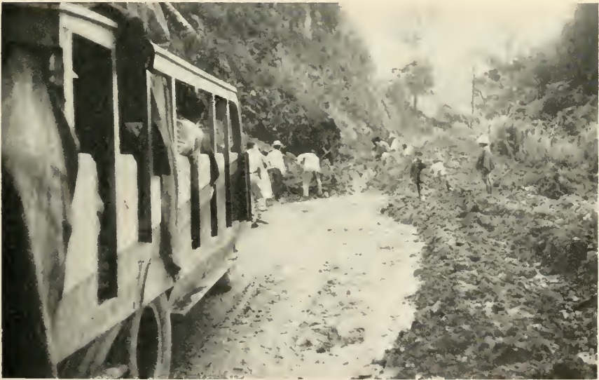
2. A bus held up by a landslide on the Garzón-Florencia road. Such occurrences mean hardships and loss of time for bus passengers, and may cause substantial losses for truckers with perishable produce.
