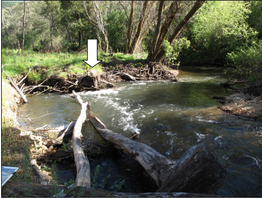
Photo 5. This bend has been eroding and now has a very unstable alignment. The floodplain on the left has been cleared of willows, including those on the bank that were providing some erosion protection (NB the stump indicated by the arrow). This bend now forms a classic 'break out point' where flood flows are free to leave the main channel and short circuit the bend. Floodplain stripping or chute cutoff development are risks at this site.
