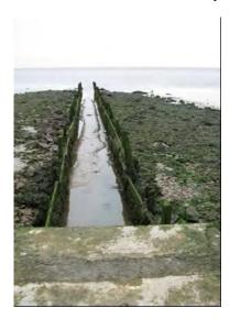
Plate 24 Post-medieval Humber outfall of Easington Clough, passing through the sea defences by means of a sluice
