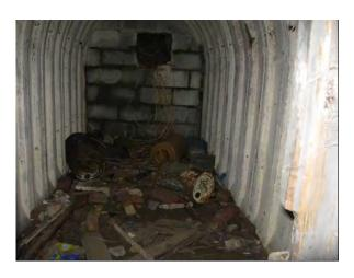
Plate 221 Side chamber formed from Stanton shelter components, WW2 observation post, North Somercotes
