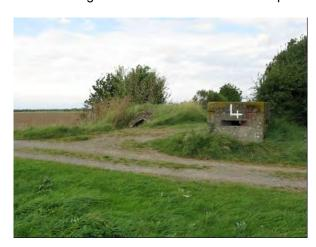
Plate 219 WW2 Observation post (right) and tunnel entrance formed from Stanton shelter components (left), Tetney
