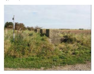
Plate 213 Triple WW2 anti-tank blocks on a single strip foundation, Holbeach
