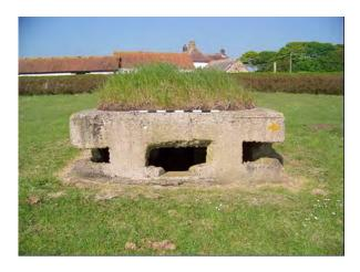
Plate 182 WW1 square pillbox with WW2 machine-qun embrasures replacing smaller original single splayed opening, Auburn Farm
