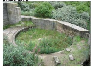
Plate 198 WW2 6-inch gun emplacement with roof removed, Light Temporary Battery, Spurn
