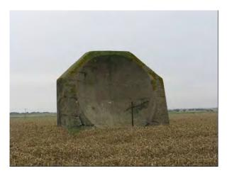
Plate 180 Scheduled interwar concrete sound mirror with surviving microphone post, Easington
