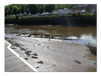
Plate 112 Late 19th-century section of patent slipway, former Whitehall shipyard, Whitby
