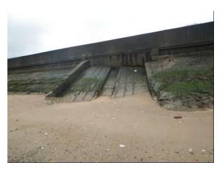
Plate 142 Disused slipway of former shipyard north of the Fish Dock, Grimsby, blocked by later flood wall
