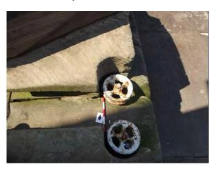
Plate 110 Cable guide pulleys within 18th-century gun embrasure forming part of 19th-century shiphandling system, West Pier, Whitby
