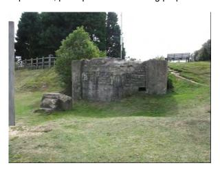
Plate 204 WW1 trapezoidal pillbox with WW2 or later additions to support observation tower for RAF Theddlethorpe air gunnery/bombing range, Skidbrooke
