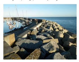
Plate 123 Modern rock armour laid against east face of East Pier, Scarborough
