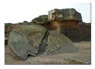
Plate 177 One of two collapsed 9.2in gun platforms, WW1/2 Godwin Battery, Easington
