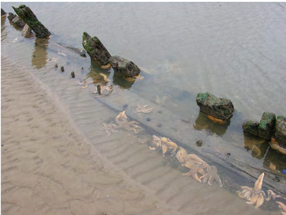
Plate 46 Detail of side planking and frame of wreck NELHER 1000/33/1, Cleethorpes, 2012 (Hugh Winfield)
