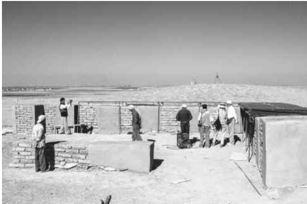
Fig. 5. Test walls, seen here during construction in 2004, were established for comparative evaluation of materials and methods of protection.
