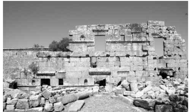
Fig. 14. The facade of the House no. 33
