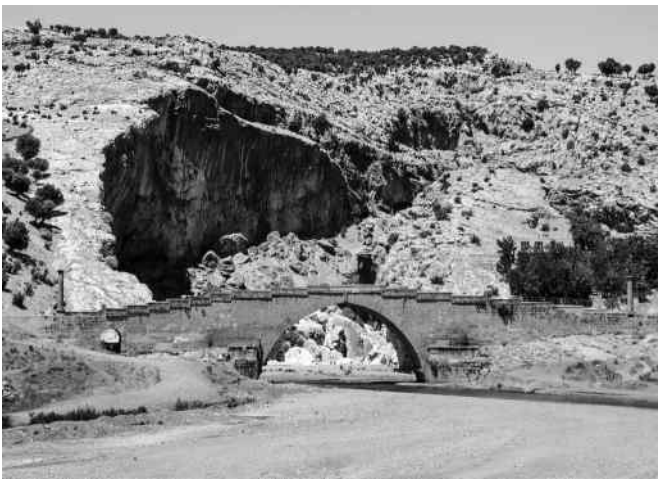
Fig. 2. Severan Bridge over the Chabinas River, Turkey; Carole Raddato from FRANKFURT, Germany [CC BY-SA 2.0 ( https://creativecommons.org/licenses/by-sa/2.0 )], via Wikimedia Commons Creative Commons Attribution-Share Alike 2.0 Generic license.
