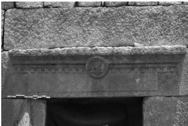
Fig. 23. Lintel with mouldings, medallions, dentil, in the House no. 2
