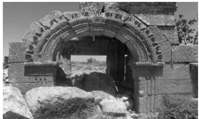
Fig. 10. The entrance of the House no.18
