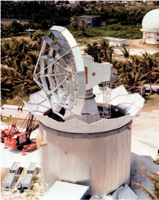
Figure 9a. The millimeter-wave radar antenna, operating at 35 GHz and 95 GHz, constructed in 1977 for the Army BMD Advanced Technology Center. This shows the millimeter wave antenna under construction (note large backup structure).
