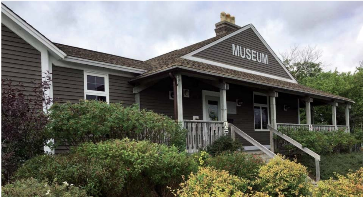
Figure 8. The main building of the Admiralty House Communications Museum.
