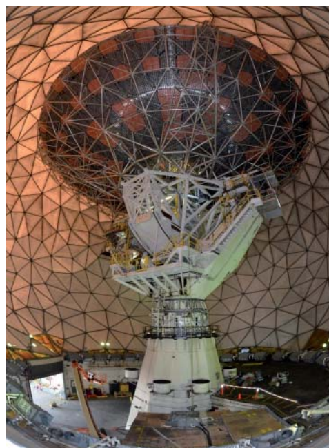
Figure 11. The upgraded antenna for HUSIR showing the new backup structure.
