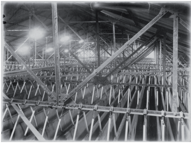
Figure 13. The plates of the massive 1.8 \mu Farad tuning air-condenser at Clifden were housed in a building measuring 350 (L) x 75 (W) x 33 (H of eaves) feet, approximately 107m x 23m x 10m, arranged in two long wings with the transmitter-receiver room sandwiched between them. It was composed of 1,800 galvanized steel sheets, each measuring 30 x 12 feet, suspended from the cross members by porcelain rod insulators in the shape of a V, as shown in the photo. (Credit: Clifden and Connemara Heritage Society).
