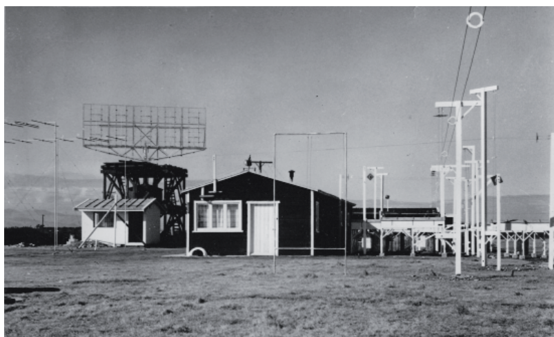
Figure. 15. Rolleston Field Station: (l-r) part of the 69 MHz meteor radiant array, GL2 rotating antenna for the meteor programme, main building housing the 69 MHz receiving-recording and winds (source: the University of Canterbury).
