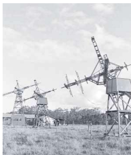
Figure 2d. Antennas of the solar interferometer at Dapto (credit: CSIRO Radio-physics Image Archive 2888-1).
