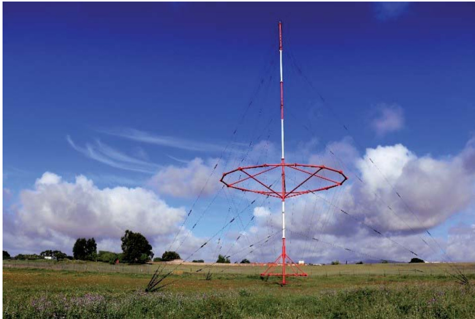
Figure 3. An HF Antenna in the ANACOM's farm in Barcarena, Portugal.
