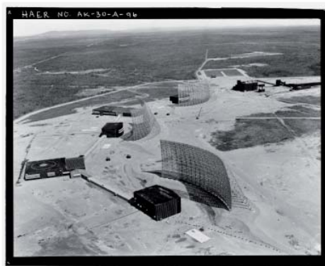
Ballistic Missile Early Warning System, Thule, 1962 (UHF band between 420 - 450 MHz) Range- 3700 km Source: Wikipedia
