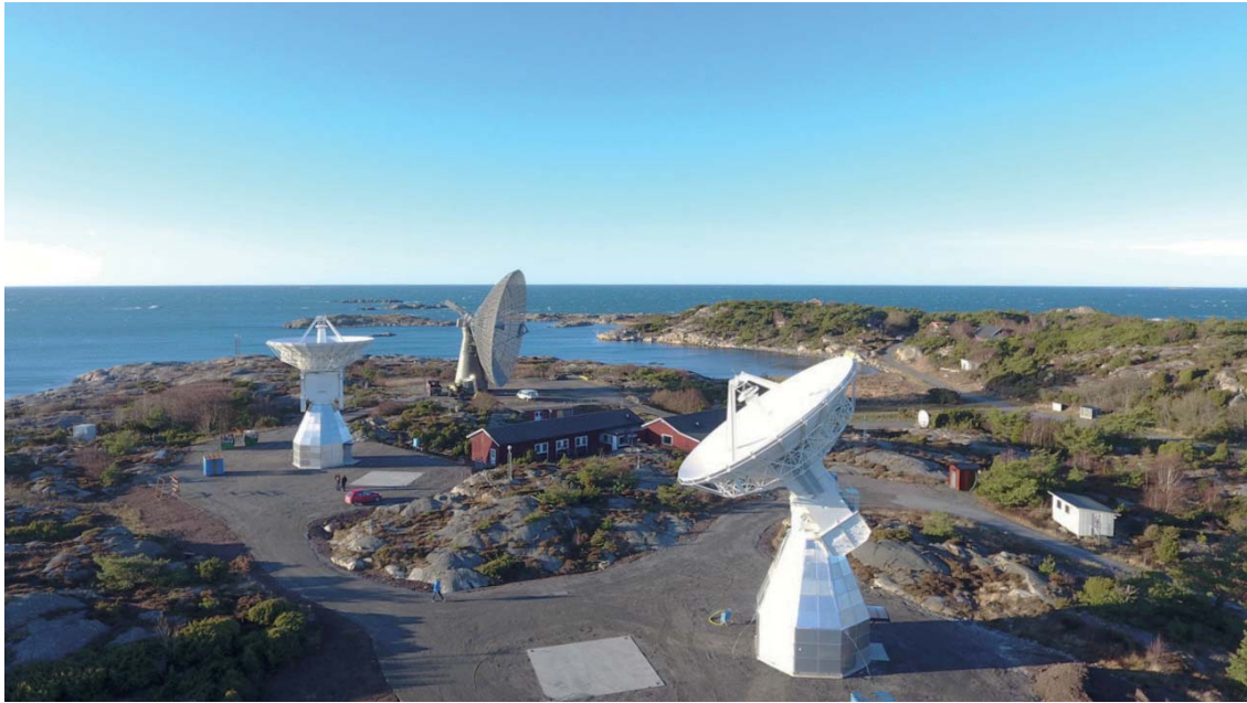
Figure 5. Antennas at the Onsala site: the grey reflector in the center is the 25 m telescope from 1963, and the two white reflectors are the 13 m twin telescopes from 2017 (photo from OSO (under CC BY-NC-SA 2.0)).
