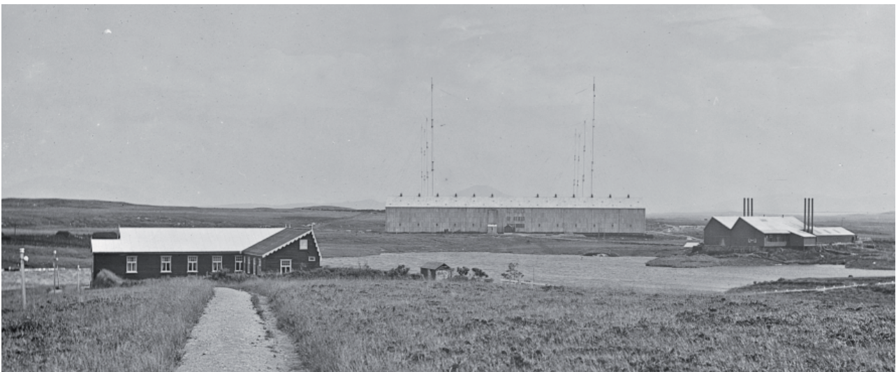
Figure 12. The original wireless station buildings at Clifden, Ireland, c. 1907, and the European endpoint of the first commercial transatlantic wireless telegraph communications link. In the center is the 350 foot-long condenser building, arranged in two long wings housing the 1800 condenser plates, with the transmitter-receiver room sandwiched between them and connected to the massive 200 ft high antenna stretching out perpendicularly to the rear of the building (barely visible). On the right is the power generation building. (Credit: Robert French, photographer; reproduced courtesy of the National Library of Ireland from the Lawrence Collection, L_CAB_04374.).
