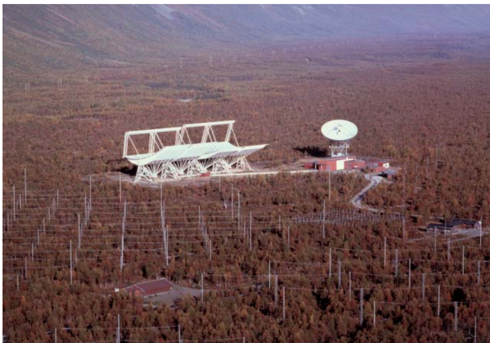
Figure 10. The EISCAT HF heating facility, in the foreground, and two incoherent scatter radars situated in Ramfjordmoen, near Tromsø, Norway. Visible are parts of three HF antenna arrays, covering 4-8 MHz, around the transmitter building housing 12 100-kW transmitters. The control building is on the right, the circular antenna is for the 933 MHz incoherent scatter radar, and the cylindrical parabolic antenna is for the 224 MHz incoherent scatter radar. (Source: Eiliv Lehren, Tromsø [8].)
