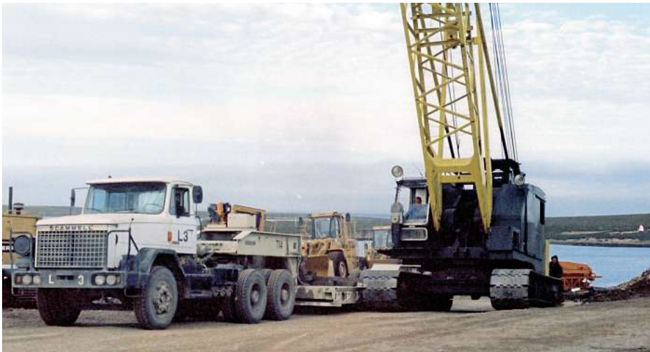
Loading an NCK Ajax 360 excavator.
