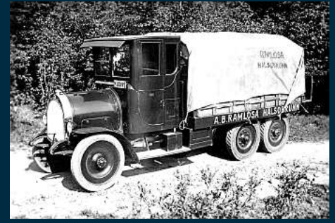
A compact little 3.5 tonne chain-drive six-wheeler from 1924. By this time Scania-Vabis was fitting double-reduction axles.
