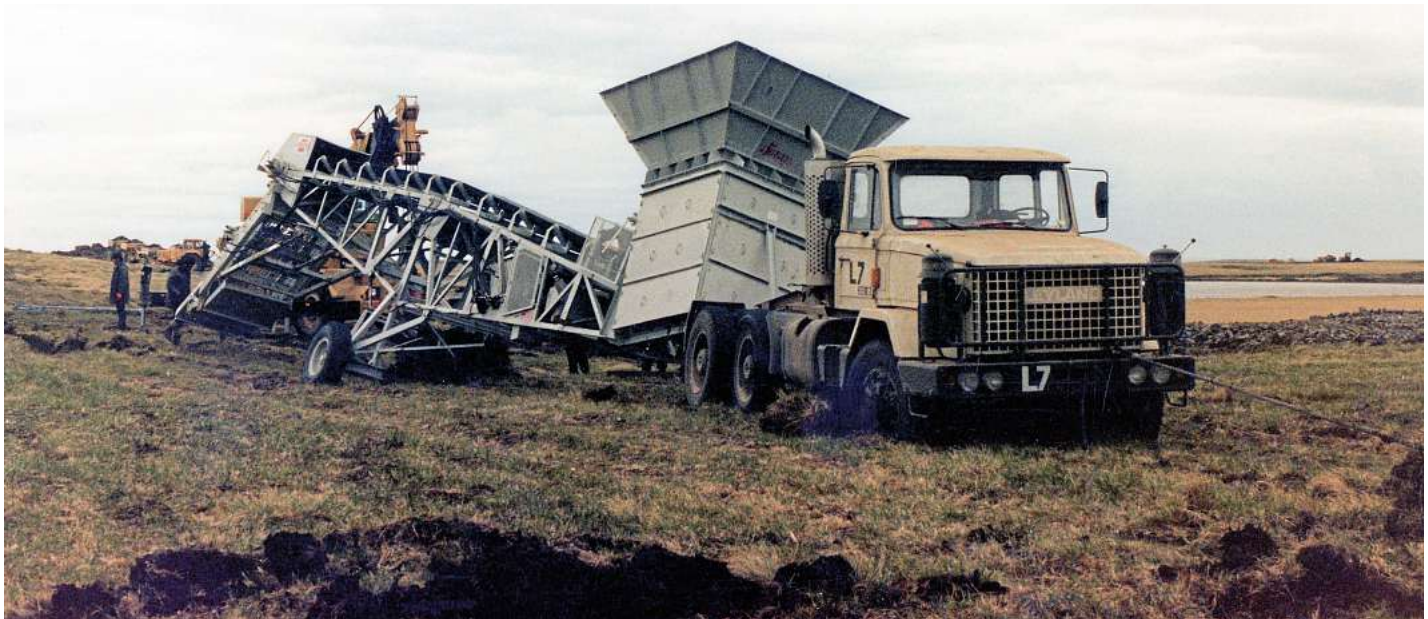
One of the Landtrains encountering difficulties in the soft peat.
