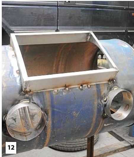
12 Here the whole thing is coming together with the window frame and arm rings fixed into place.
