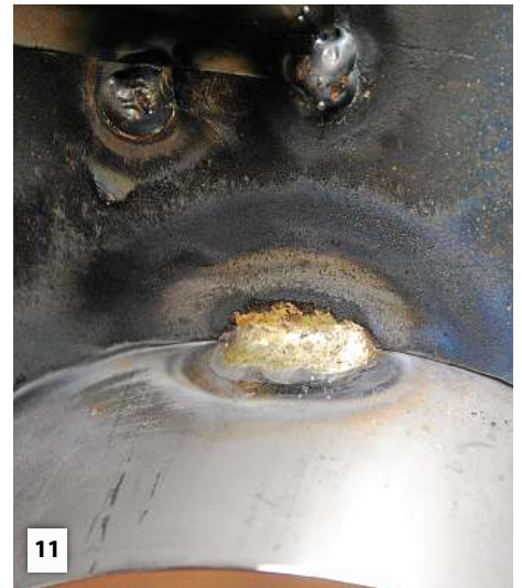
11 The arm rings which are made of stainless steel were brazed into the barrel in several places; if they had been mild steel these too would have been welded in.
