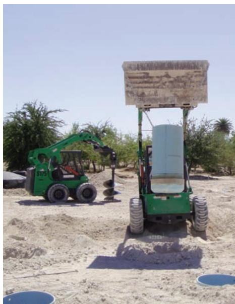
Setting the lysimeters into the holes at UCR. Researchers will check leachate collection equipment from each plot and identify 8 plots for use in the research commencing in the summer of 2009.
