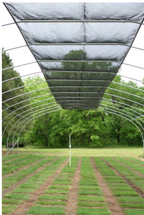
A 75% black woven shade cloth was installed above the plots to provide shade in the middle of the day.
