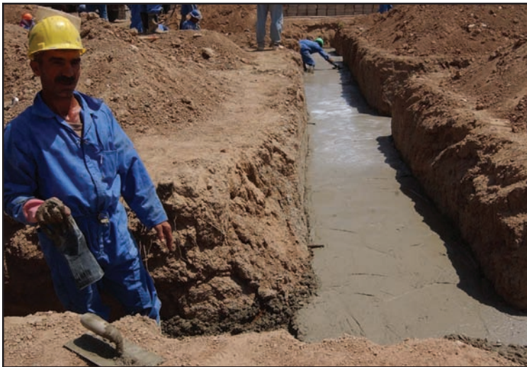
Figure 92. An Iraqi laborer finishes the concrete footings for an Iraqi Army barracks complex at a new Iraqi Army base near Kirkuk, Iraq.
