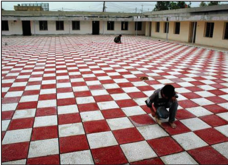
Figure 89. Iraqi subcontractors lay concrete tiles at a school play yard renovation project outside of Irbil, Iraq.
