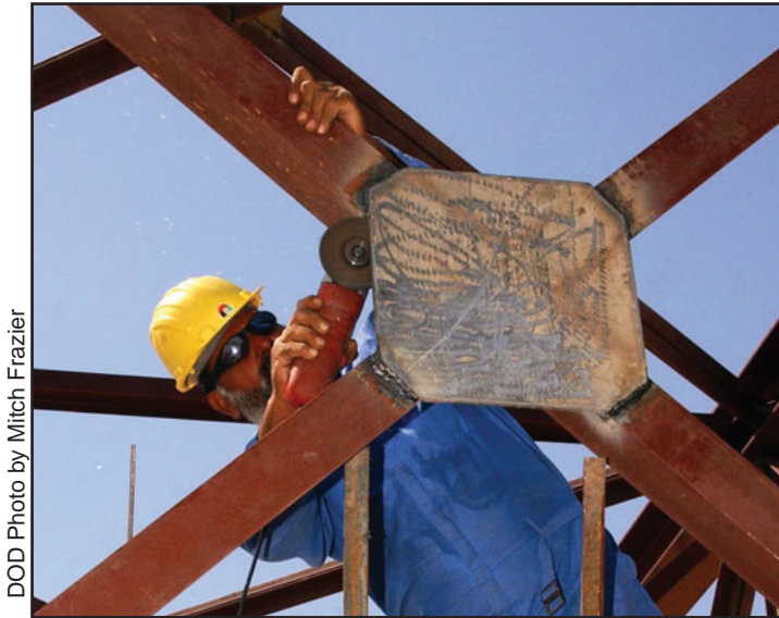
Figure 133. An Iraqi laborer grinds a plate on a metal support structure at a military training base in eastern Iraq. The structure supported a water storage tank that will soon supply the base with clean water.
