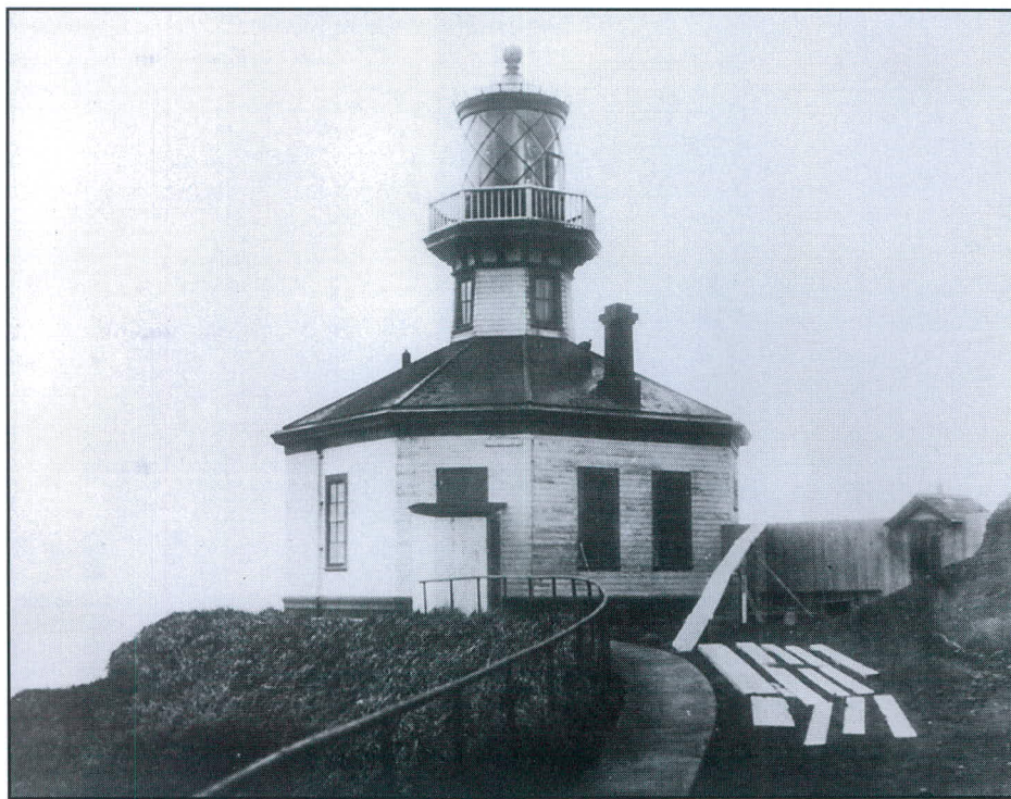
The Scotch Cap Lighthouse shortly after completion in 1903. This octagonal design was also used for the Cape Sarichef Lighthouse located at the other end of Unimak Pass. Note the diagonal astragals of the lantern room. The Lighthouse Service started using this British design after the turn of the century. The dwellings were located several hundred yards away as seen on page 27. U. S. Lighthouse Society photo.
