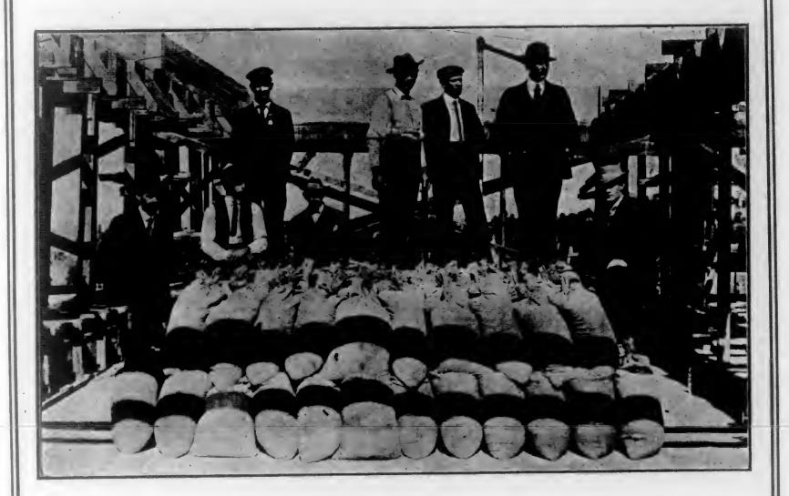
ONS of sacks filled with sand were placed on the floors of the Bixby Hotel, causing a super-imposed load of 240 pounds per square foot. This load is six times the load for which these floors were designed, and is equivalent to the weight of three tiers of heavy men packed together as closely as possible, and one tier on top of another.
