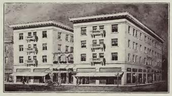
Montgomery Hotel, San Jose. An All-concrete Structure, Reinforced with Deformed Steel Bars. This Building Is Nearing Completion on Utill Cost Close to \$200,000 William Building, Architect
