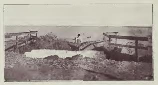
A Pair of Twin American Ingot Iron Culverts, Being Installed in Kern County, Cal.
