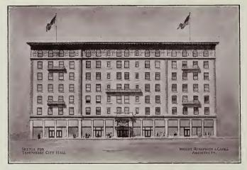
Temporary City Holl, San Francisco, Controct for the Concrete Work Alone Amounted to Nearly \$200,000, Foundations, Curtain Walls, Floars and Roof Are All of Concrete Wright, Rushforth & Cohill, Architects
