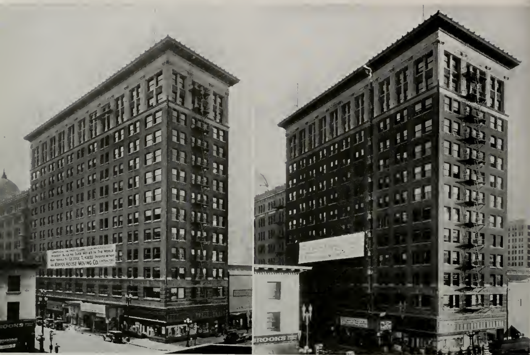
Commercial Exchange Building, Los Angeles. Picture on left shows building before cut in two; Photo on right shows appearance of building after rejoining the two sections.
