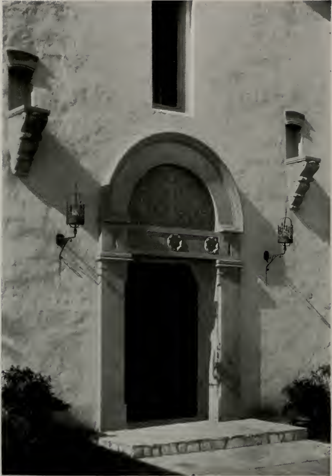
DETAIL OF ENTRANCE, CHURCH OF ST. ANTHONY, GARDENA, CALIFORNIA
