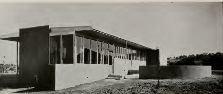
THE N. KOBLICK RESIDENCE, ATHERTON. RICHARD NEUTRA, ARCHITECT
