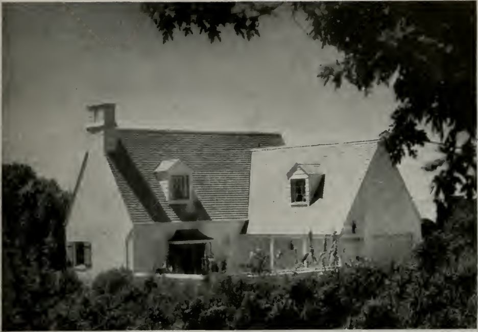
RESIDENCE OF MR. AND MRS. RAYMOND BOWERS, BERKELEY Frederick L. Confer, Architect
