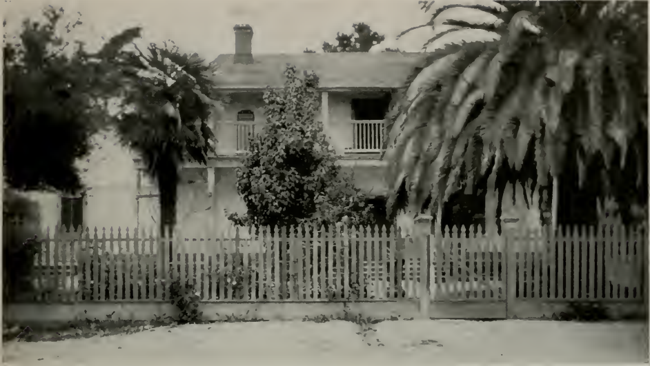
TYPICAL OLD TYPE OF HOUSE IN MONTEREY, CALIFORNIA Photograph by Archie T. Newsom
