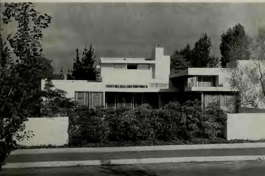
RESIDENCE FOR MR. AND MRS. G. G. BUCK, LOS ANGELES R . M . Schindler, Architect
