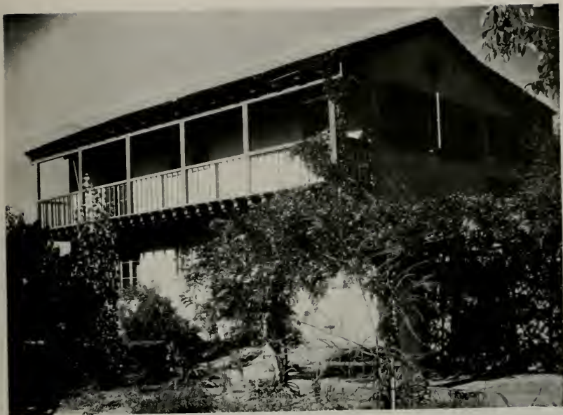
RESIDENCE FOR T. FENTON KNIGHT, LA CANADA, CALIFORNIA Henry Carlton Newton and Robert Dennis Murray, Architects
