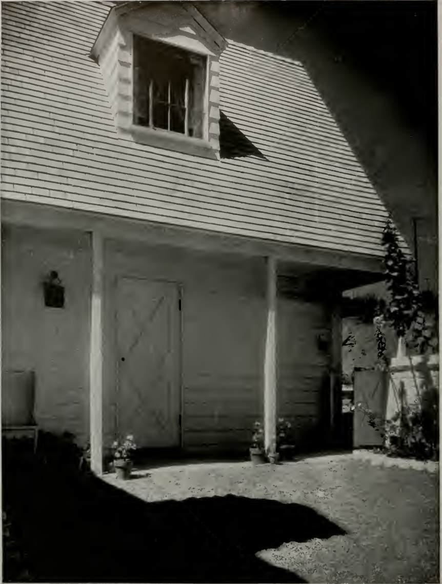
ENTRANCE COURT, RESIDENCE OF MR. AND MRS. RAYMOND BOWERS, BERKELEY, CALIFORNIA FREDERICK L. CONFER, ARCHITECT
