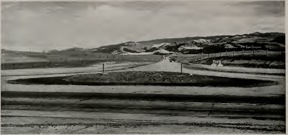
CROSS AND CAMPANILE will mark this intersection of the new road to the Mission town of San Juan Bautista with the Prunedale cutoff, San Benito County, California (Courtesy California Highways and Public Works)
