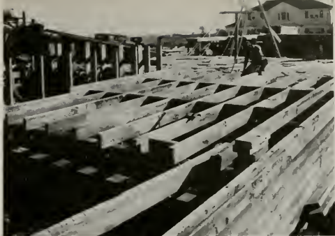
Pressure treated lumber for home of Dr. John L. Pomeroy at Brentwood being placed.
