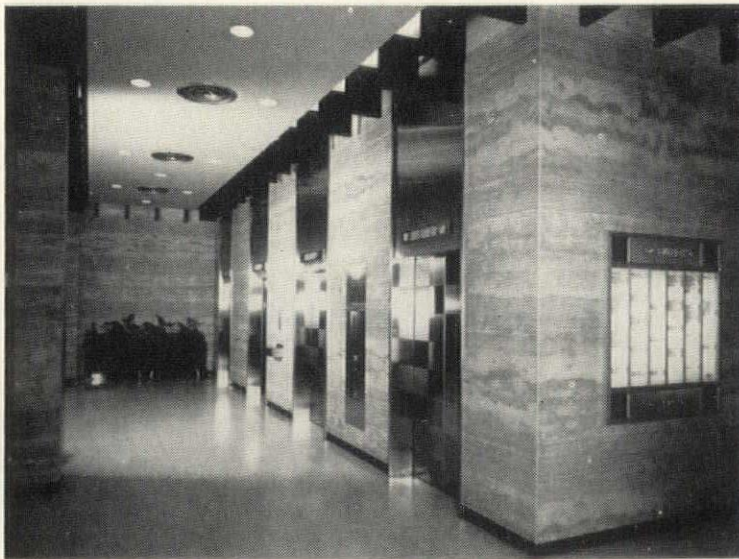
730 Baker Building Installation of Quarry Travertine Marble Baker Associates Incorporated
