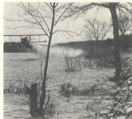
Bentonite was placed by plane along the dikes during the flood danger (Photo courtesy Minneapolis Tribune).
