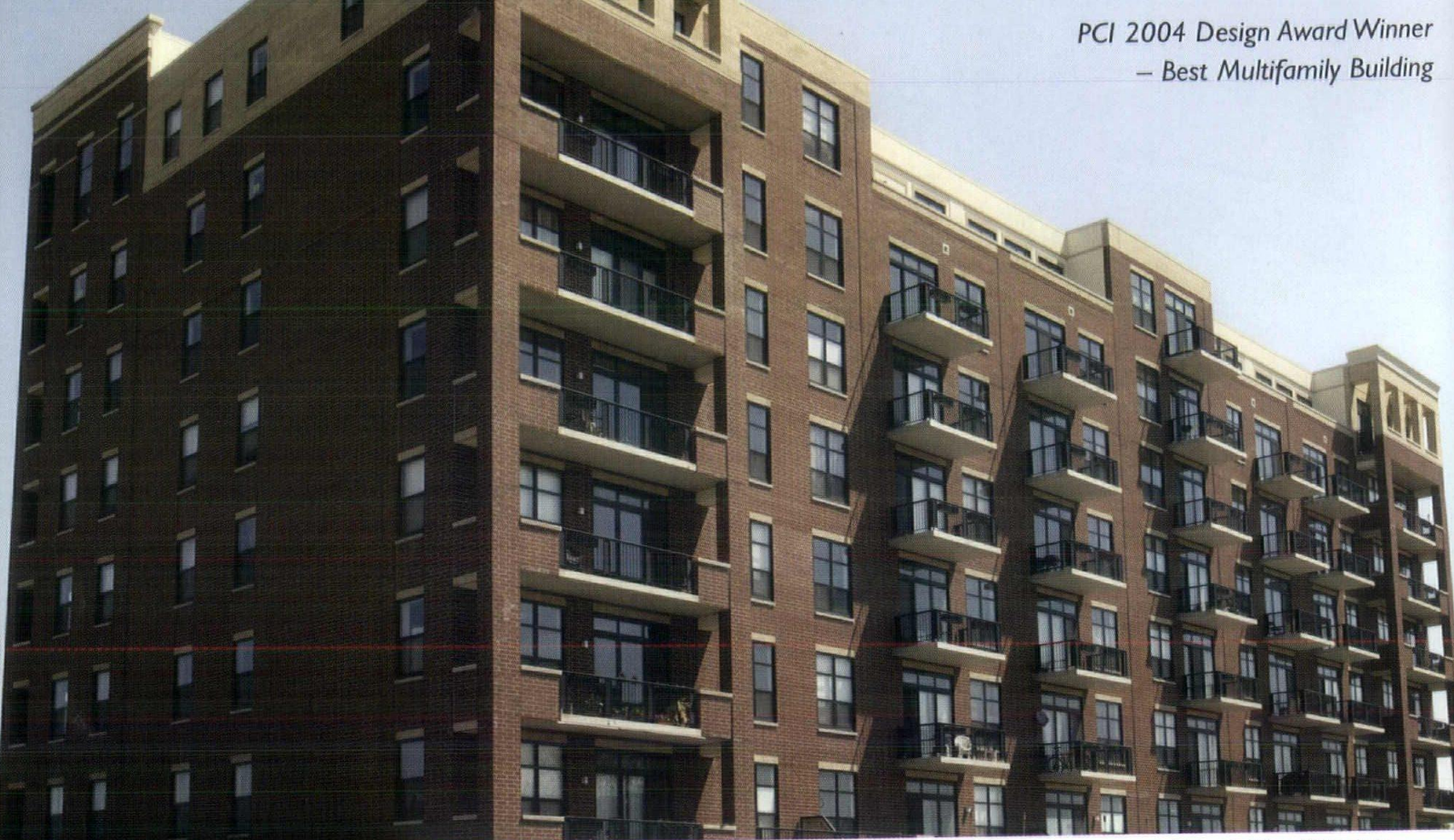
University Village Midrise Lofts Total Precast Structural Frame Chicago, IL
