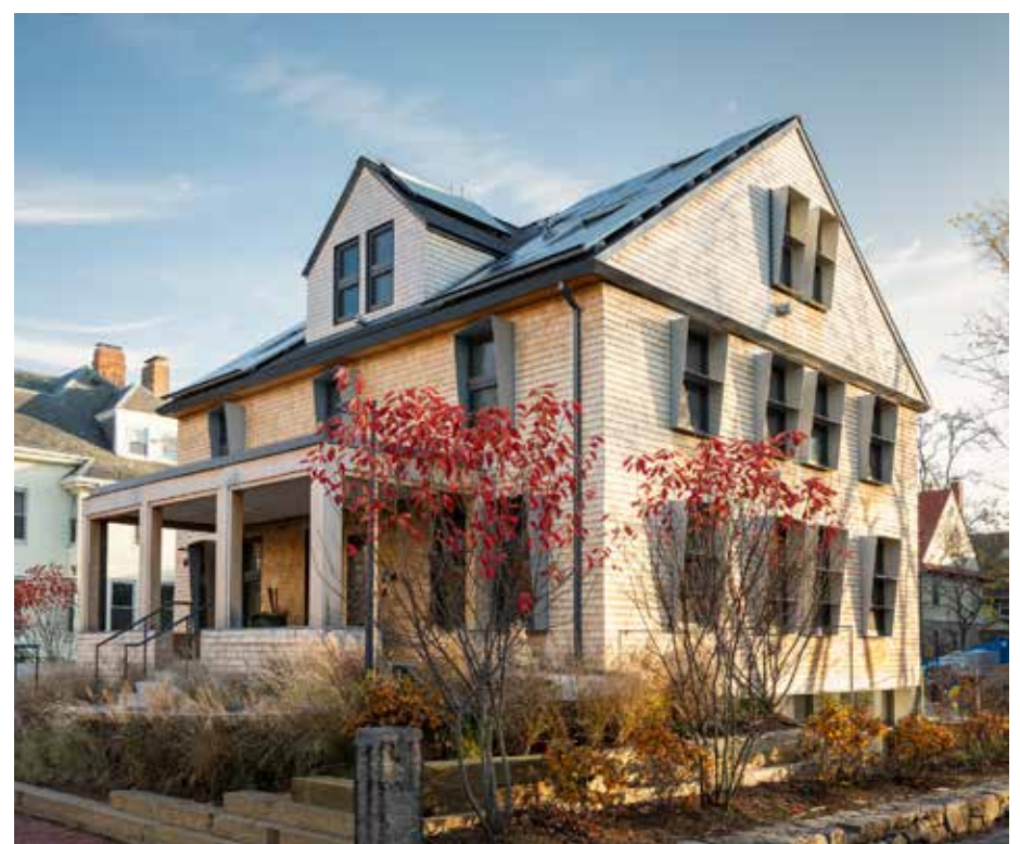
Top: Snøhetta poured a concrete floor slab that passively absorbs and releases heat. Above: Sculptural solar shades and solar panels were added to the house's exterior.
