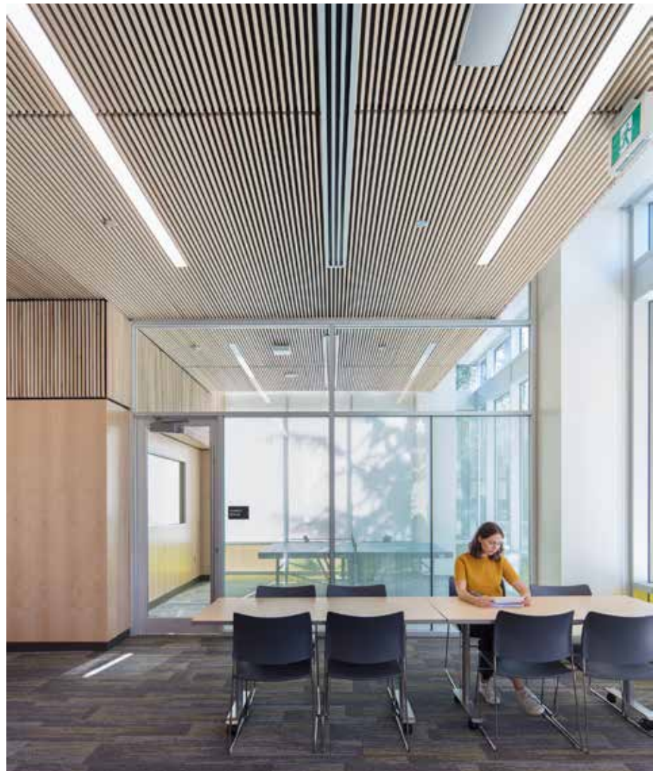
The project features custom maple veneer paneling by JSV Architectural Veneering & Millwork as well as slatted albus wood ceiling panels by Linea Ceiling & Wall Systems.
