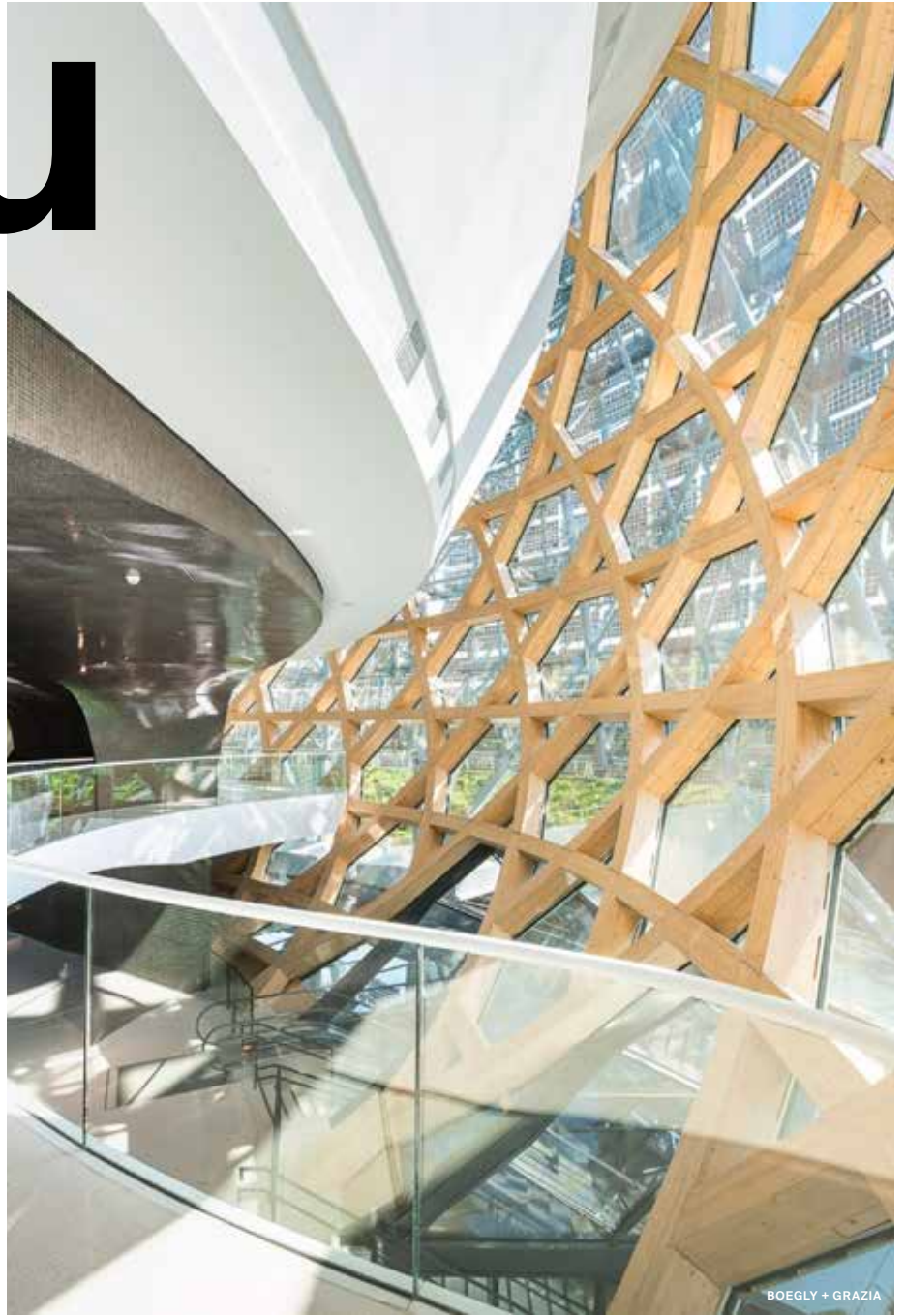
La Seine Musicale, a performing arts center in the Paris area, is wrapped in a timber and glass skin.
