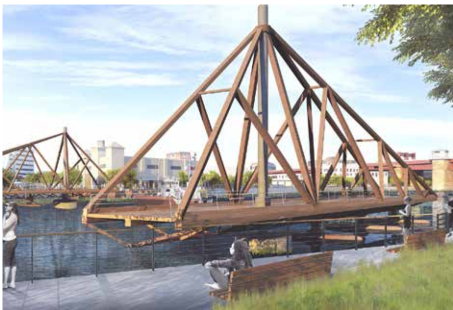
The timber bridge proposed by CRÈME/Jun Aizaki Architecture & Design is intended to be lightweight and relatively inexpensive, and pivots open in the middle to allow larger vessels to pass through.
