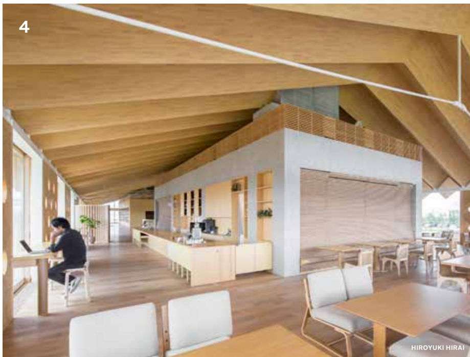
3. The Swatch buildings compose the world's largest timber project. 4. For a new hotel in Japan, SBA created a lightweight folded timber roof.
