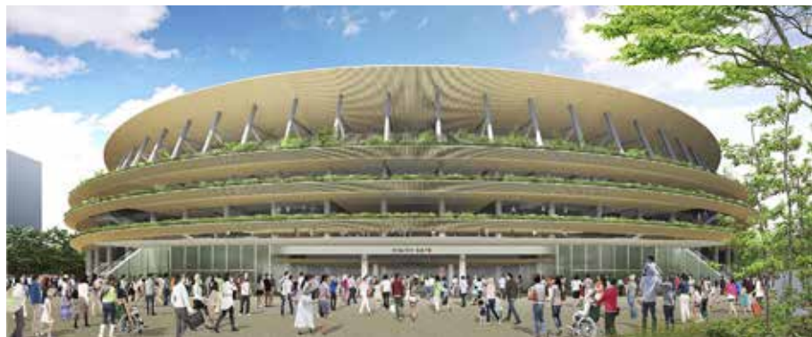
Top: The center of the stadium has been left open both to allow in natural light and to create a chimney effect where hot air can escape. Middle and Above: The stadium is ringed with breezy colonnades, a reference to Japan's historic timber pagodas.
