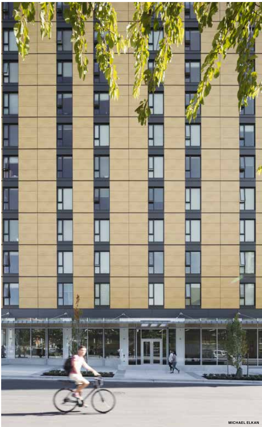
The 18-story Brock Commons tower is a monument to mass timber, containing 464 CLT panels, including repeating facade panels manufactured by Centura Building Systems and Phoenix Glass.
