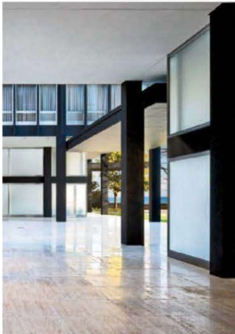
Back-of-house areas are once again concealed by panels of sandblasted glass, as they were when the buildings were completed in 1951.
