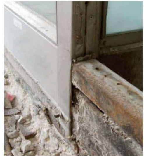
The plaza's poor drainage caused deterioration of the lobby storefront, especially at the base.
