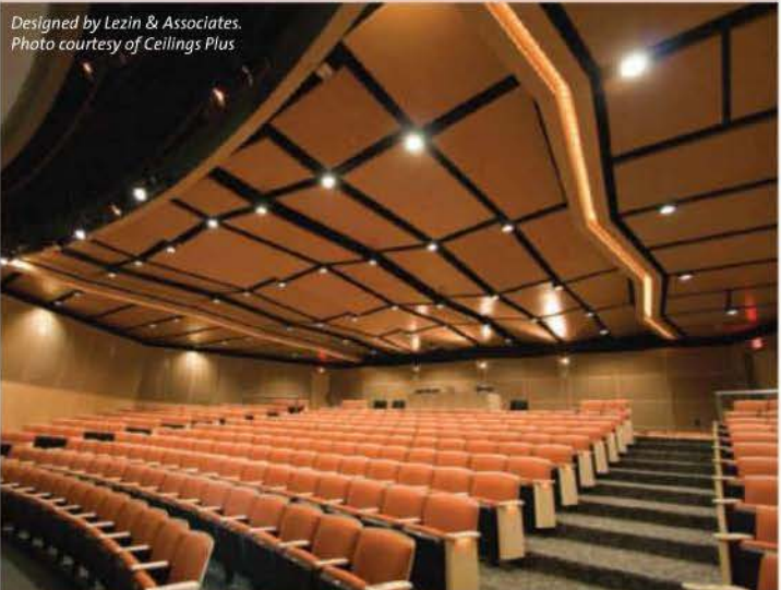
Wood wall and ceiling panels at Pitzer College, Claremont, CA auditorium are lightweight and perforated to provide acoustical control.
