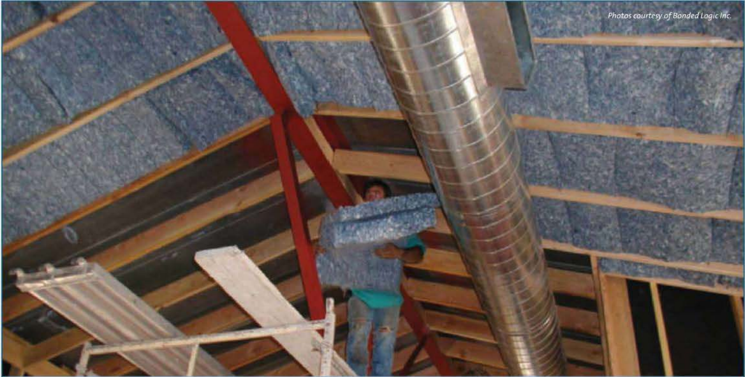
Insulation has greater resistance to conductive heat losses compared to other building materials.
