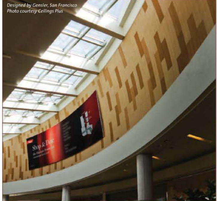
Designed by Gensler, San Francisco Photo courtesy Ceilings Plus Panels are curved in both the X and Y axes to create a gently curving wall in the Westfield Galleria, Roseville, CA.
