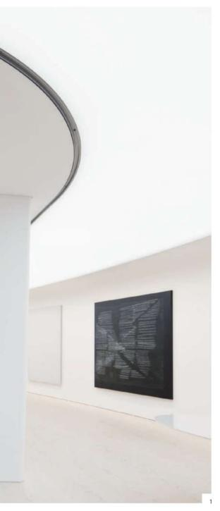
1. In a New York City loft building, the architects designed the space where an art collector lives to have a flowing, light-filled backdrop for his art. LED lights above two layers of stretch translucent fabric give a luminous quality to the ceiling. The existing steel columns clad in terra-cotta are filled out with preformed glass-fiber-reinforced-gypsum elements, as are other curved components in the space.
