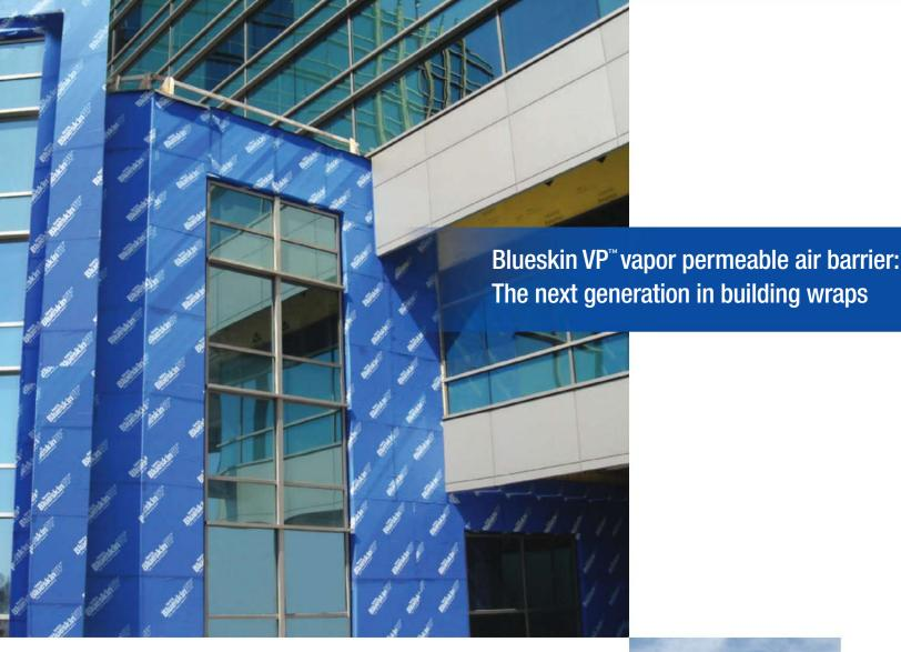
Another first from Henry® Company, the leader in Building Envelope Systems®, Blueskin  $VP^{\mathsf{TM}}$  is a fully-adhered membrane system that functions not only as a water resistant barrier and rain barrier, but also reduces uncontrolled air leakage caused by various conditions, such as stack effects, wind effects and mechanical air handling effects.
