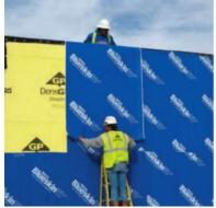
Self-adhering membrane eliminates fasteners that leave holes in the building envelope.
