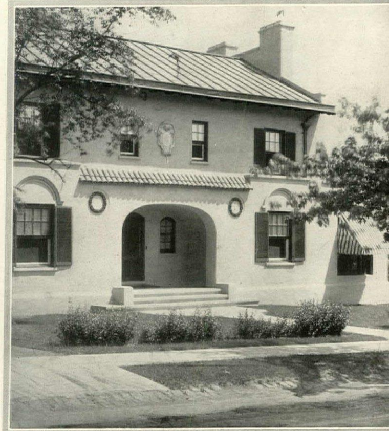
The judicious use of glazed terra cotta decorations in color make an effective ornamentation for the cement house. The indented entrance porch and the arched window panels also help
