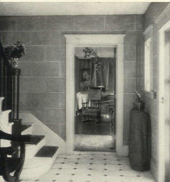
The vestibule walls are soft brown, the plaster laid directly on hollow tile. The marble floor is from an old dismantled house
