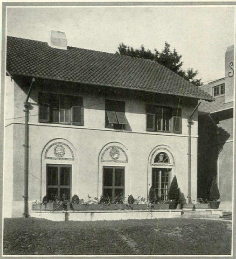
The factors which here mitigate the concrete nakedness are the wide overhanging eaves, the small window and door panes, the indented arches and mosaic work. Mann & MacNeille, architects
