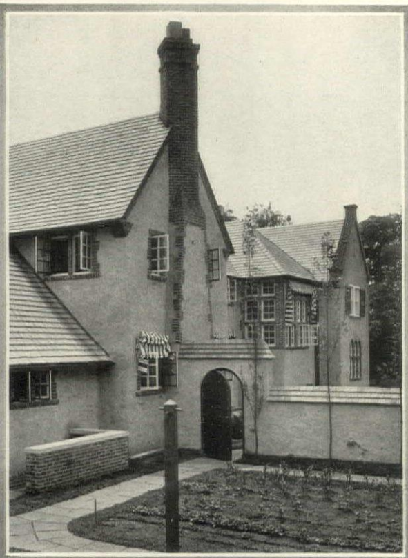
In this country house, of which Edmund B. Gilchrist is architect, brick trim has been attractively combined with rough concrete finish
