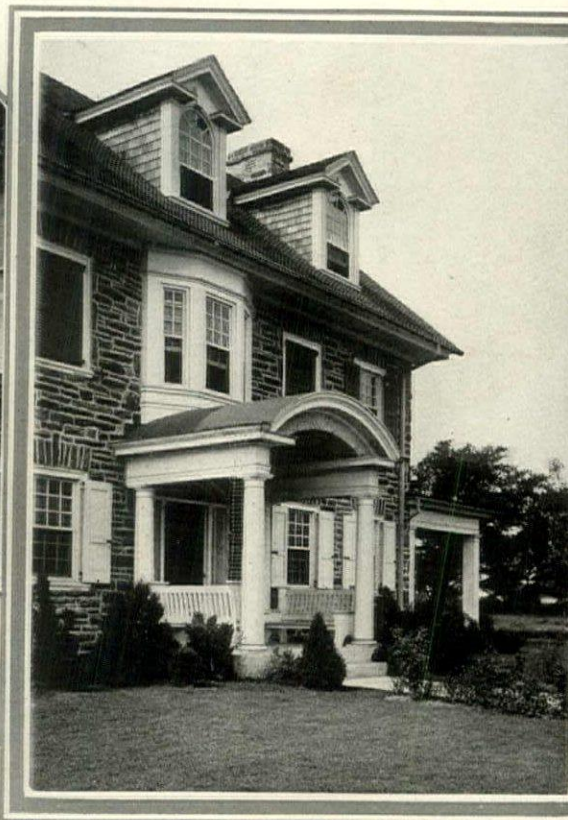
The Roman Doric column has been used here. Its characteristic is its proportion—the height being eight times the diameter, thus assuring, under usual conditions, a graceful appearance
