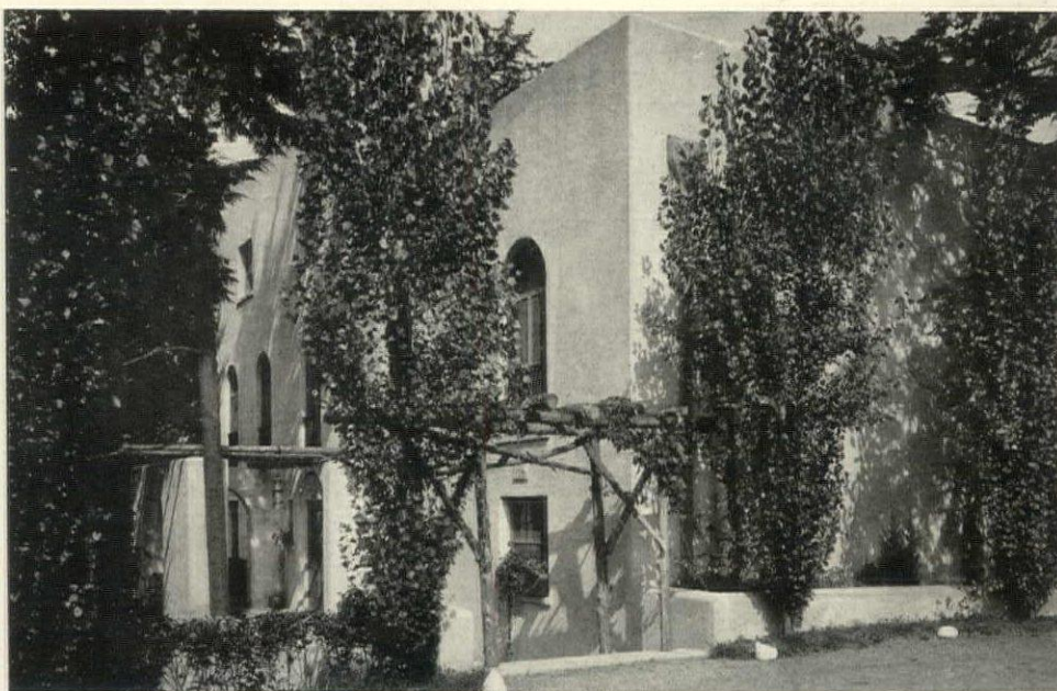
Hollow tile was used—6,500 of them put in place by three masons and seven helpers in twenty-seven working days. The whole was then covered with cement. There is one chimney to serve the four flues
