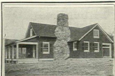
Stained with Cabot's Creosote Stains Brookie & Hastings, Architects, Philadelphia
