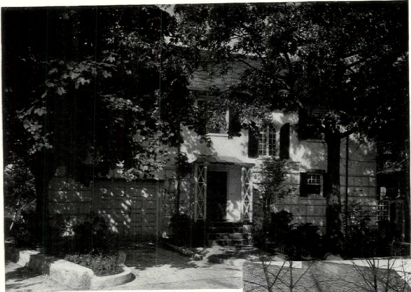
FRONT BEFORE AND AFTER
