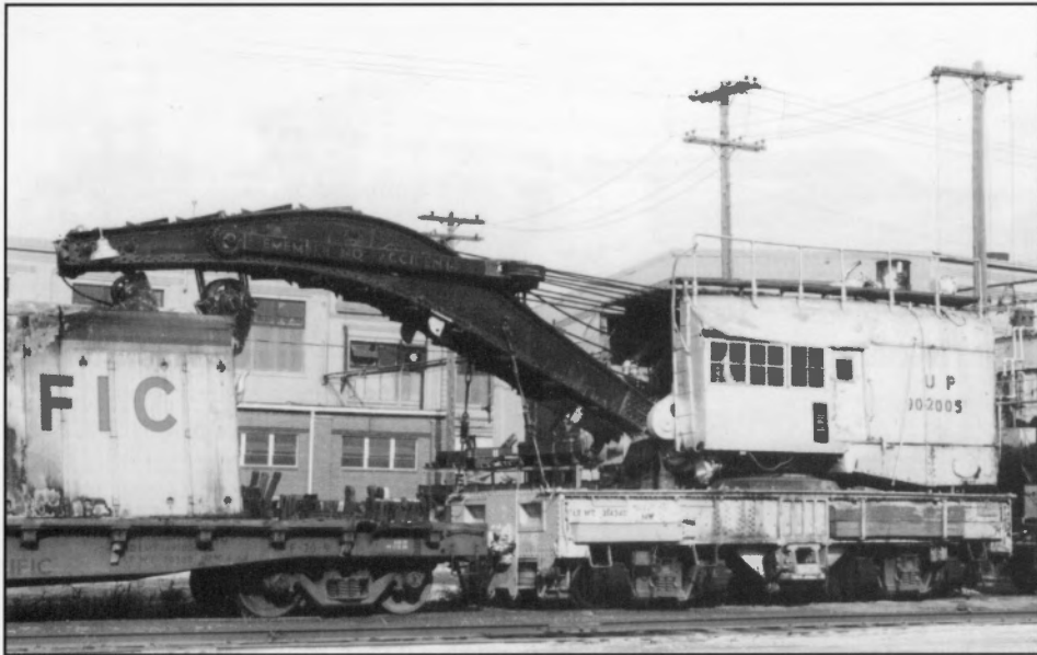
120- ton 902005 was built for the Oregon Short Line by Bay City in 1913. Converted from coal to oil in 1952, it had plain bearings and was not self-propelled. Before retiring in 1975, it was assigned to Glens Ferry, Idaho and Albina and Hinkle, Ore. When this picture was taken at Omaha on June 26, 1975, it had just returned from clearing up a wreck, as evidenced by the engine hood on the boomcar. The walkway on the roof was constructed from GP 9 handrails J.R. Quinn, collection of John C. LaRue Jr.
