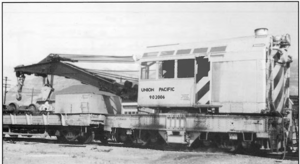
Wrecking derrick 902006 was donated to the Canyon County Museum at Nampa, Idaho, after it was retired in October 1979. This car was the last steam powered wrecking derrick owned and operated by the Union Pacific. Built by the Industrial Brownhoist Corporation in 1917 for the Oregon Short Line, it had a capacity of 150 tons. Note the larger windows for better viewing compared with 903037, which was built only seven years earlier. Black chevrons on the door are unusual. H.N. Proctor, J.C. LaRue Collection.
