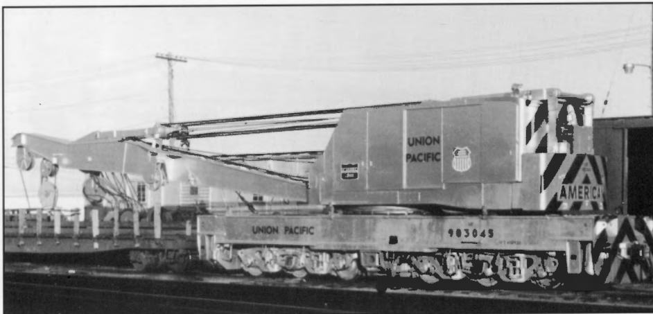
Four 250 ton units purchased in the late 60s and early 70s by the UP. Built in 1969 by American Hoist & Derrick, the car has the normal steel construction, diesel power, roller bearings. It was photographed at Rawlins, Wyo., on July 3, 1970. This series of cars has three outriggers on each side, one in the center and one on each end, and the two three-axle trucks span the length of the car. F.H.Worsfield, collection of John C. LaRue Jr.
