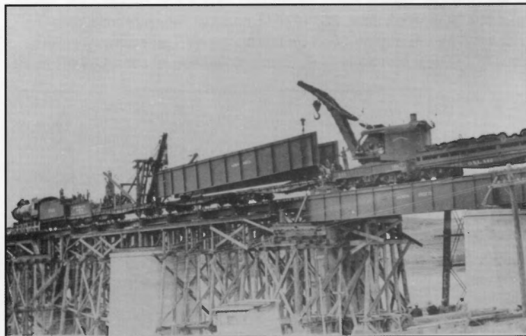
Wrecking derrick 902006 was donated to the Canyon County Museum at Nampa, Idaho, after it was retired in October 1979. This car was the last steam powered wrecking derrick owned and operated by the Union Pacific. Built by the Industrial Brownhoist Corporation in 1917 for the Oregon Short Line, it had a capacity of 150 tons. Note the larger windows for better viewing compared with 903037, which was built only seven years earlier. Black chevrons on the door are unusual. H.N. Proctor, J.C. LaRue Collection.
