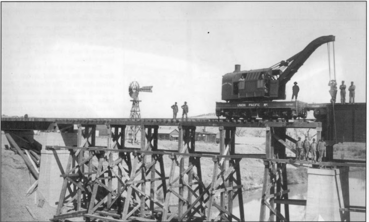
A view of 02797 at Fort Steele, Wyo. in 1901. This 40 ton derrick was constructed in 1899 by Industrial Works and weighed 140,000 pounds. It was 24' 2" long and had a steel underframe and wood superstructure and burned coal. The car was renumbered to 03052 in 1918 and retired in 1952. The wrecking derrick was working in conjunction with wrecking derrick 02801 to install the girders on the bridge. The bridge crews typically had a derrick car on each end of the girder to lift the beam up and off from the flatcar before placing it in position on the concrete piers. Stimson photo Wyoming State Historical Society.
