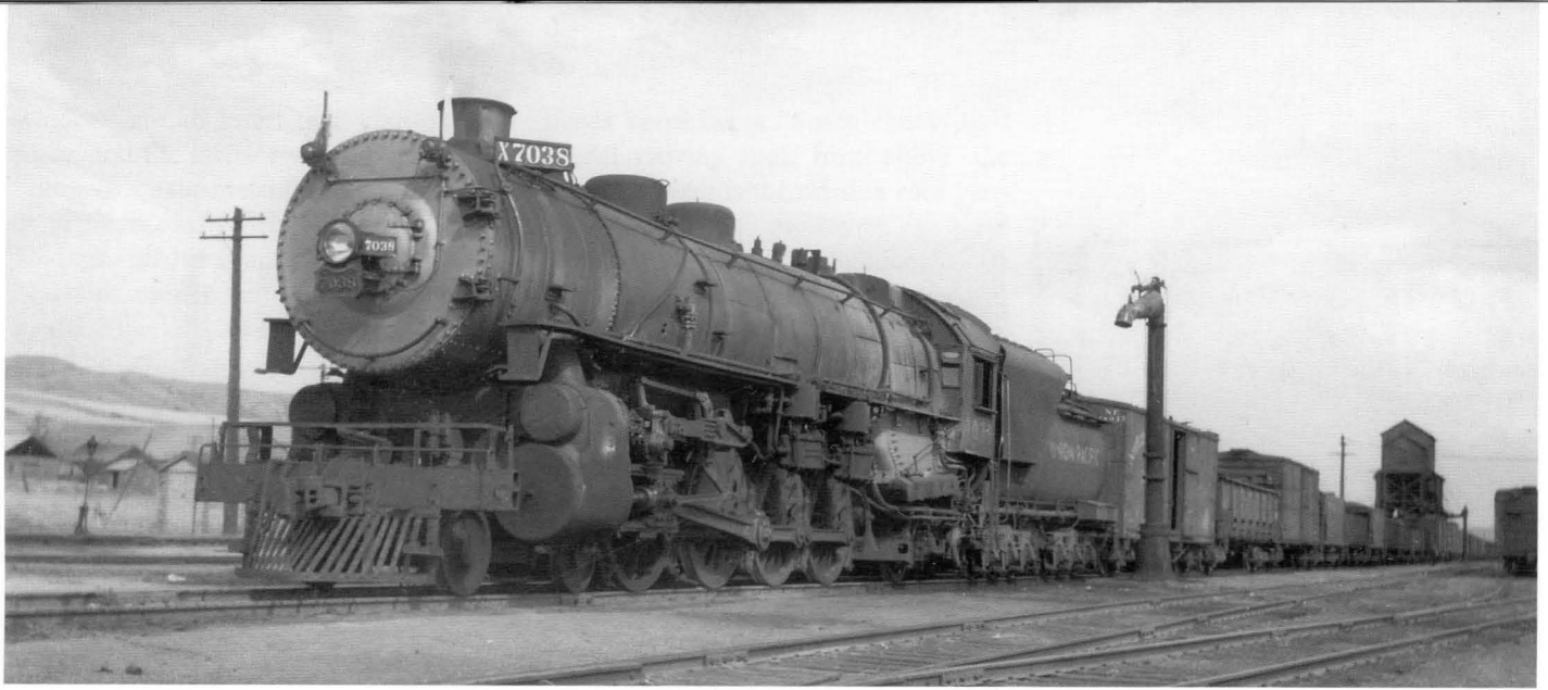
UP Mountain class 7038 sits at Cache Junction, above, with an extra freight on August 22, 1940. Built in 1922, these versatile locomotives were used regularly on both passenger and freight trains, all across UP's far-reaching system. Train 553, right, is the Cache Junction to Preston passenger train, shown here prior to departure at the Cache Junction depot, with two cars in tow on May 30, 1938. The 568 is subbing for the regularly scheduled motor train. The unusual smoke stack treatment on the 568 is a spark arrestor that consisted of numerous rods installed across the stack. Timetables show Train 262 as a daily Ogden to Pocatello time freight, it is shown, below, leaving Cache Junction powered by a 2-10-2. Although the even number on the train's indicator denotes this as an eastbound train, this train is actually traveling north through Cache Junction, before eventually heading south to Ogden. -Three photos, Emil Albrecht, Don Strack collection
