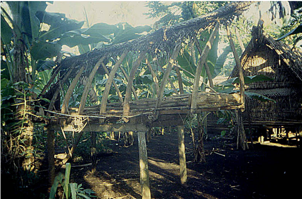
From 1996: Iwa yamhouse framed with trees designed to last from one year to the next, though the structure is re-enclosed every year before it is ritually loaded with new prestations of yams. Pandauns leaves or woven coconut fronds form the usual covering.
