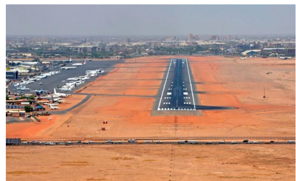
Figure 4: Khartoum international airport runway
