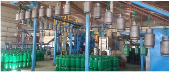
Figure 34: Factory for LPG cylinders
