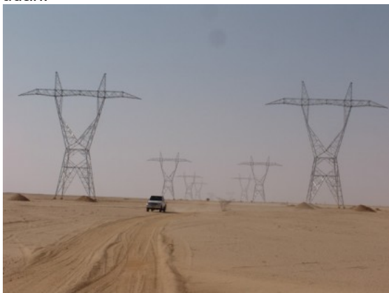
Figure 10: Electricity transmitter in Merowe Dam
