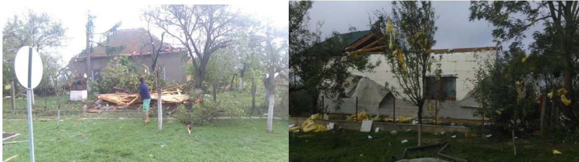
Effects caused by the violent storm of Recas - September 2017.
