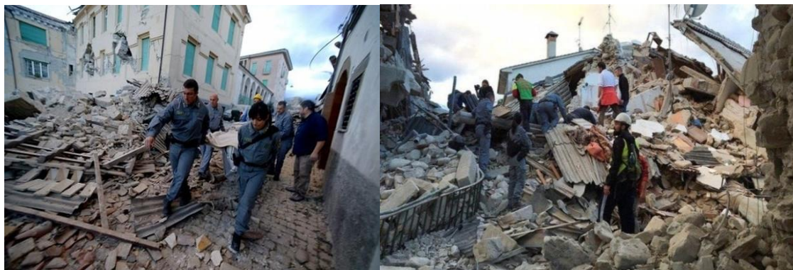
Consequences of earthquakes in urban areas. Source:Google - earthquake images.
