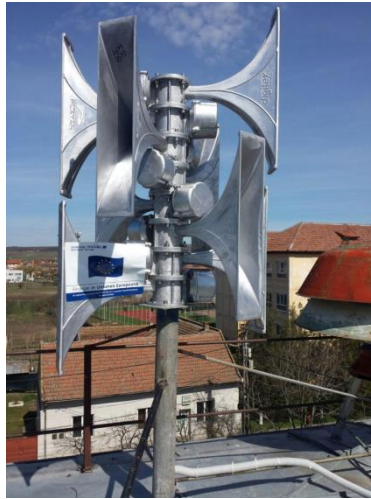
High power electronic siren, with 4-8 loudspeakers.
