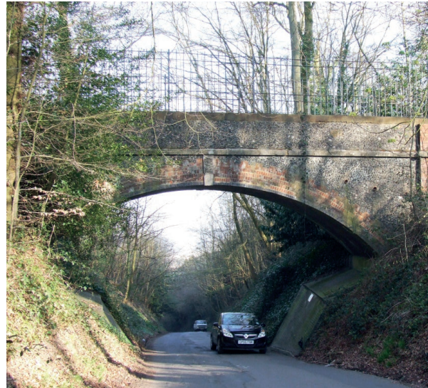
Trosley Towers Bridge in April 2009
