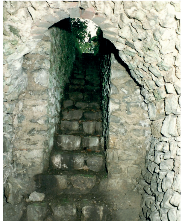
Tunnel at Malling Abbey
