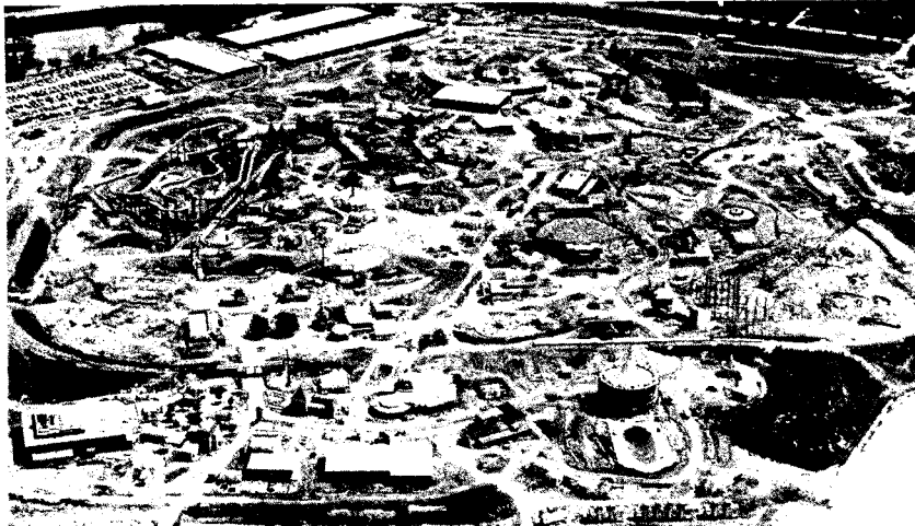
GREAT AMERICA FROM AIR — This is an aerial view of Marriott's Great America theme park under construction in Gurnee. Most obvious "landmark" is $1 million double decker carousel, "The Columbia." Proceeding clockwise from carousel one can distinguish five themed areas that are taking shape to form Marriott's Great America. These areas are: Orleans Place, a realistic depiction of the Old South in the mid-1800's; Yankee Harbor, an early 19th century New
