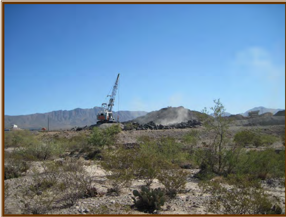
Photo 11. View of crane east of action area, facing east.
