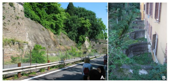
Landslides along the left side of the Tiber river valley, due to slow movement of the Pliocene clays . A. The external wall of Villa Sciarra collapsed in 1990. B. The edifices at the base of Monteverde hill have been built with horizontal arcs to prevent the effects of decompression of the overconsolidated Pliocene clays.
