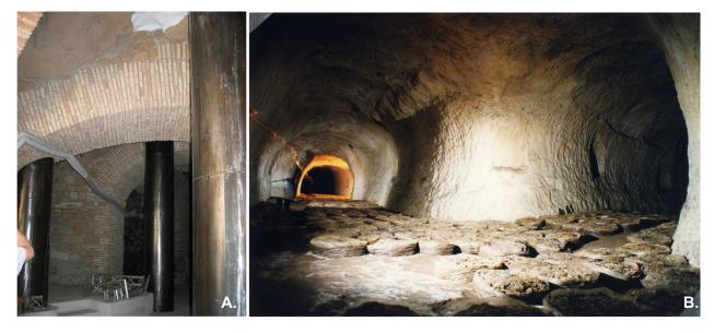
A. Tunnel excavated in the Tufo Lionato at Monteverde originally to extract building stones, have been re-inforced and longly used. Note also the vertical pole-foundation which have penetrated the tunnel from overlying constructions; B. Underground cavities used for mushroom-growing.
