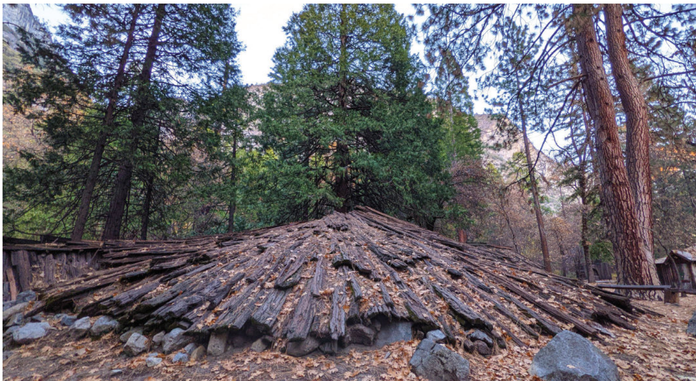
The sweathouse of the Miwok people was used for ceremonial and health purposes by the men of the village. Incense Cedar poles provide the framework of this structure that was then covered with layers of buckbrush, wormwood, pine needles, cedar bark, and soil.
