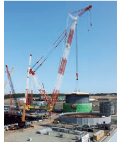
Installation using a large rotating crane
