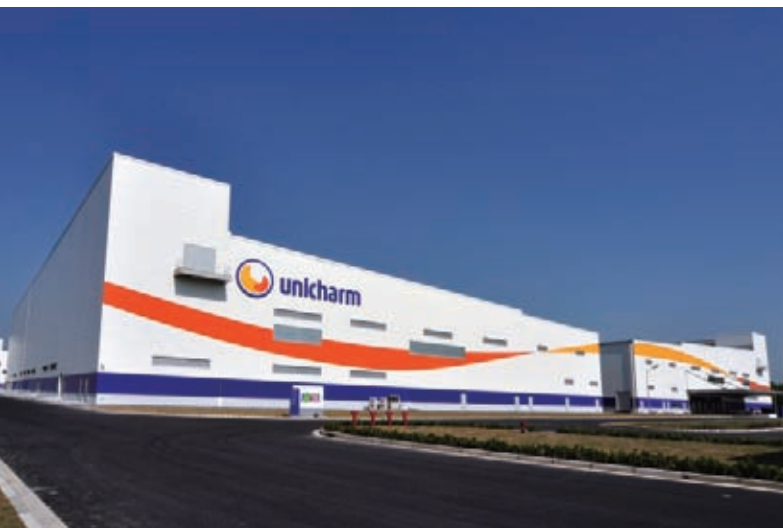
Unicharm Corporation Shanghai Factory
