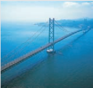
Akashi Kaikyo Bridge
