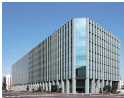
Eastnet Building II
