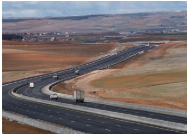
East-West Motorway, Algeria
