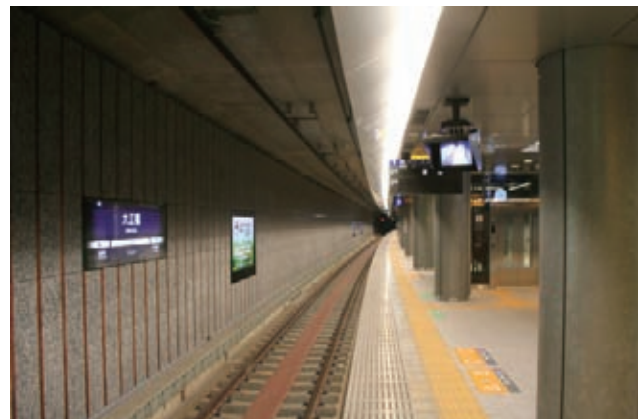
Oebashi Station, Nakanoshima Line
