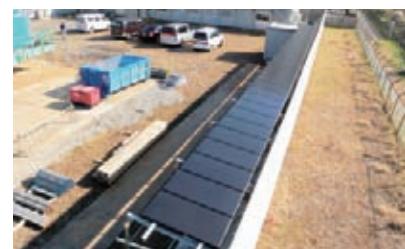
Solar panels used at construction sites
