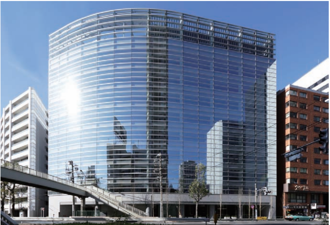
Aoyama Kajima Building
