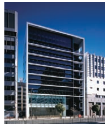
Akasaka 2-Chome Building
