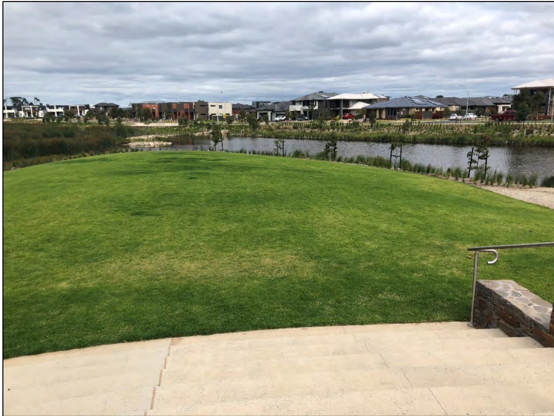
Figure 2 Expected look of a Sediment Basin within a Retarding Basin. Source: SWS
