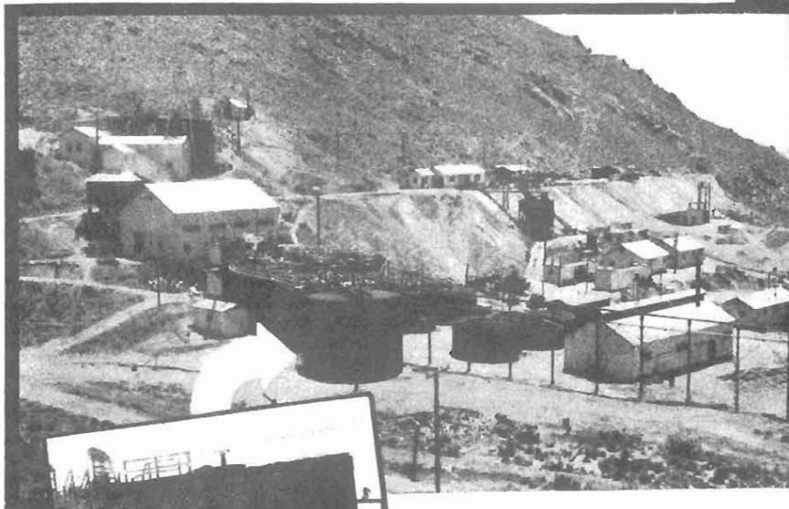
Cactus Mines: Dorr Washing Thickener in foreground, conventional C. C. D. system directly behind.
