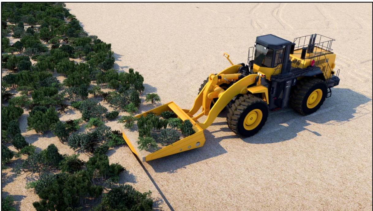
Figure 4: VDT excavation (sod removal) method
