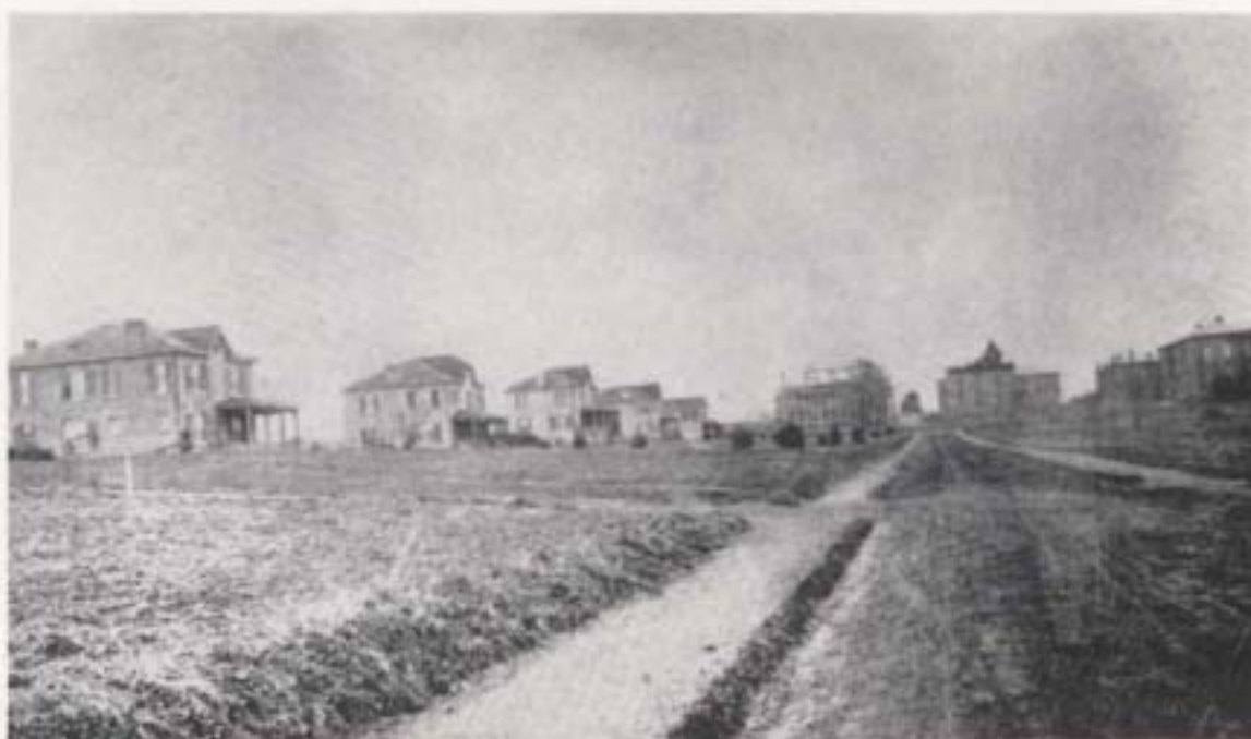
FACULTY ROW IN 1901. Note the Military Building—formerly the Y. M. C. A. Building—under construction and "the pretty grounds." Many of these houses have been moved several times to allow for expansion of the physical plant.
