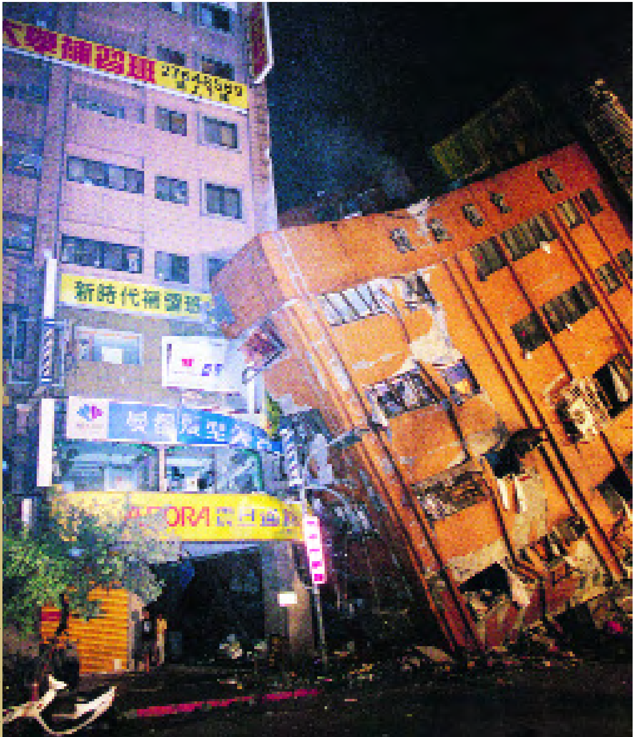
Collapsed buildings after an earthquake in the Taiwan Province of China. LO TSUNG HSIEN/UNEP/STILL PICTURES
