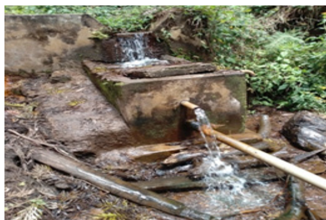
Plate 16: Intake inside Nzai Water Tower
