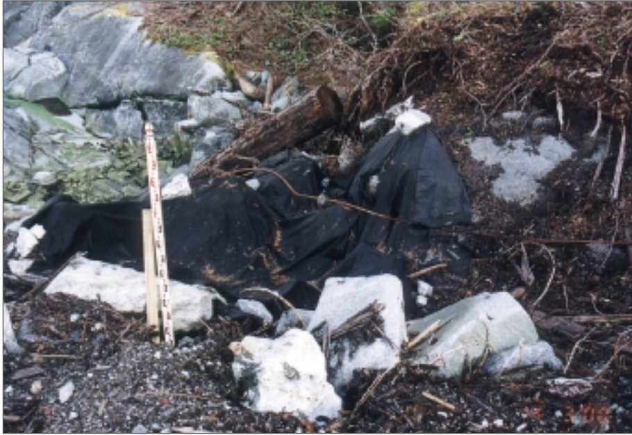
Photo 35: Water bar, fitted with geotextile, separating foreshore from operating surface; Verney Passage dumpsite (March 2000).
