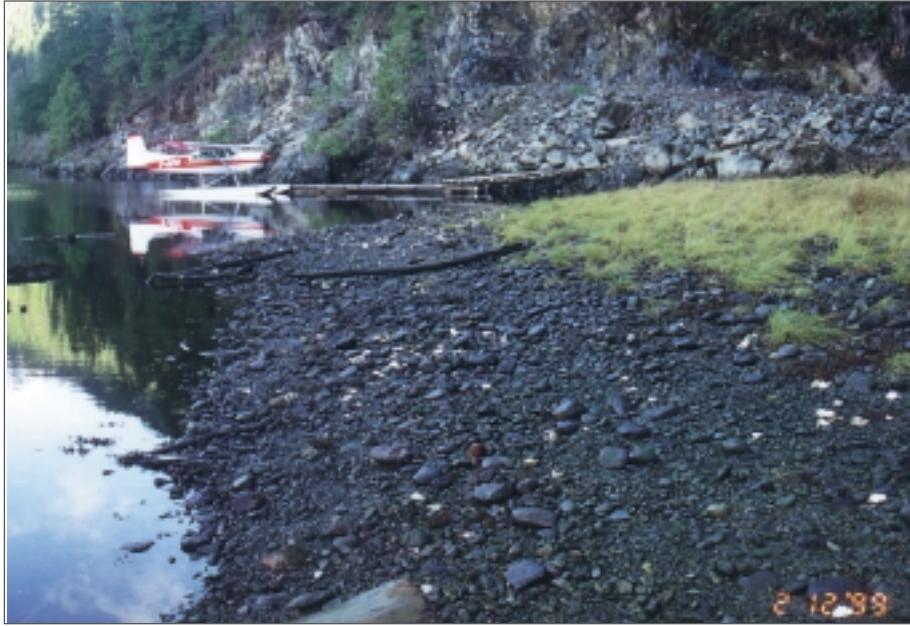
Photo 50: Brand Creek log dump, Effingham Inlet; “reference” foreshore in foreground, dock and upslope running surface in background (December 1999).
