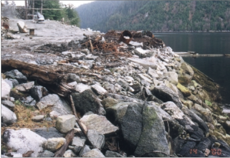
Photo 27: Foreshore and intertidal fill; Trip Creek dumpsite (March 2000).
