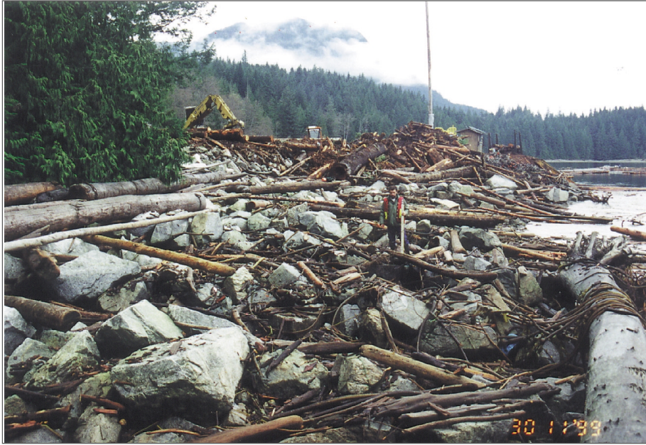
Photo 64: Debris washed up on compensatory rock “fingers”, Knox Bay log dump (November 1999).
