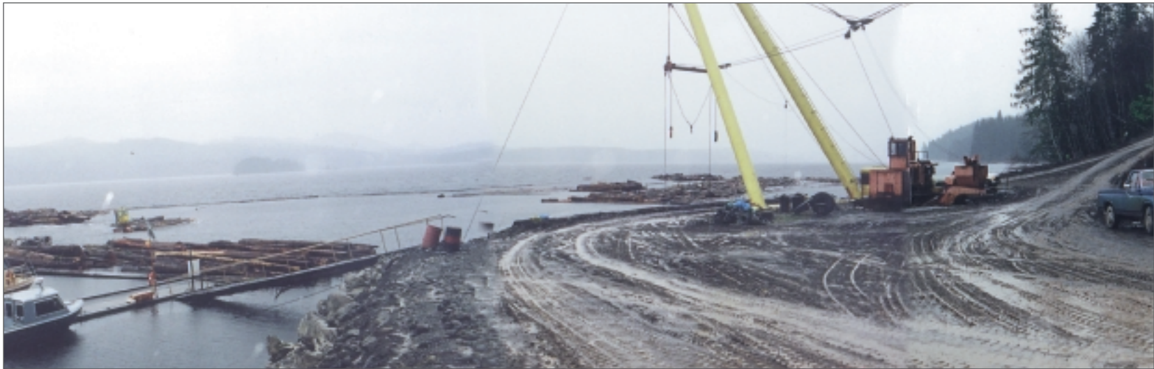
Photo 71 : Michelson Point dump, running surface, view westward (November 1999).
