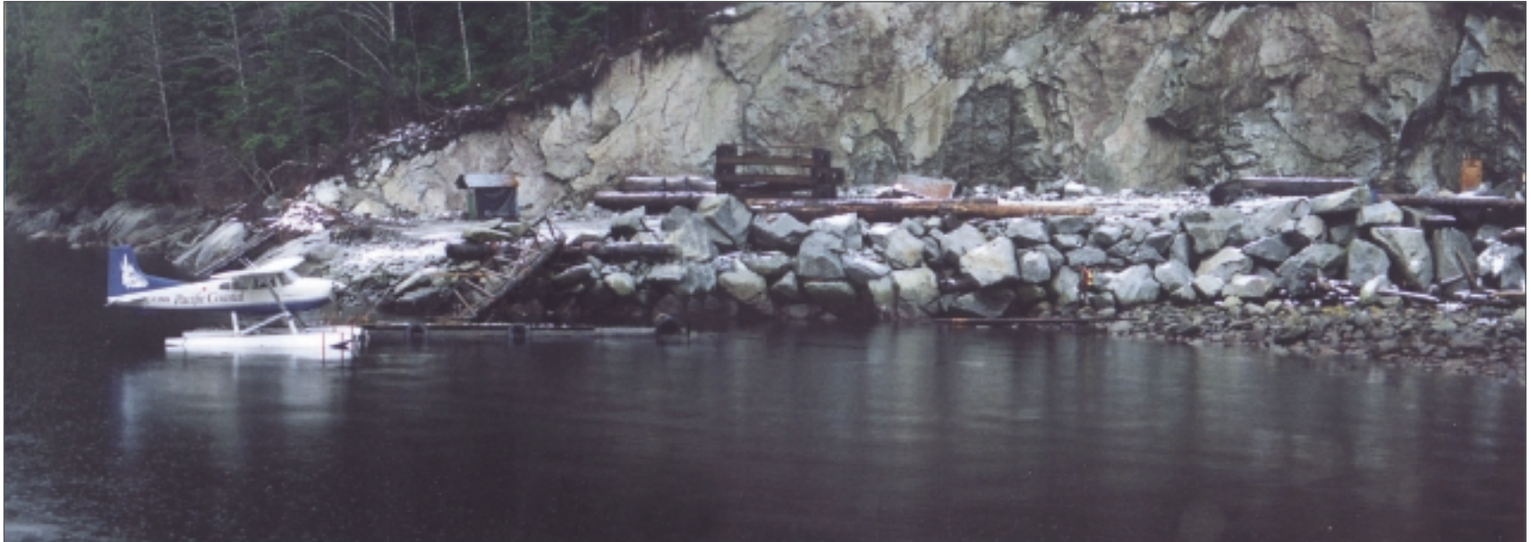
Photo 3: The Fog Creek dump was blasted from steep bedrock, then shot rock used as fill (December 1999).
