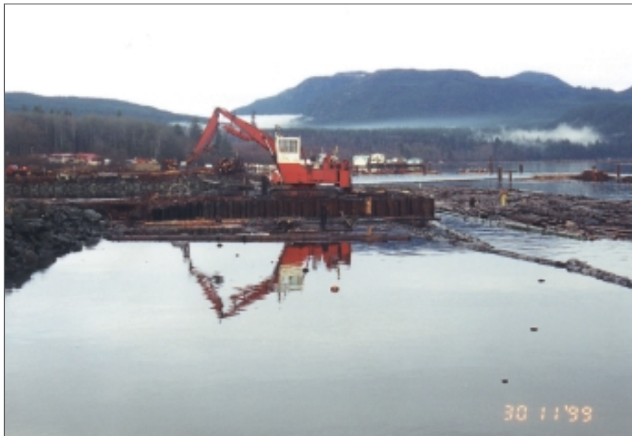
Photo 61: Crane dewatering site, Campbell River Fibre, Menzies Bay (November 1999).
