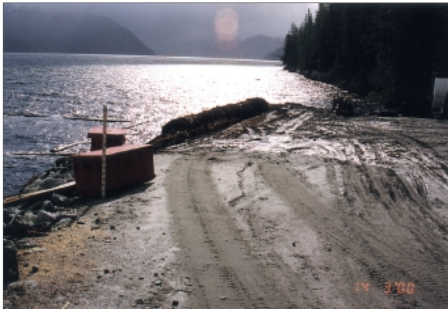
Photo 17: East Gribbell Island log dump, running surface with little pooled water (March 2000).
