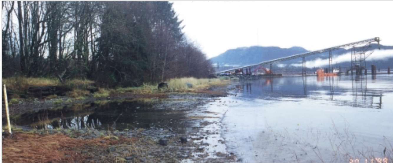
Photo 58: Habitat compensation site with crane dewatering and conveyer facilities in background, Campbell River Fibre, Menzies Bay (November 1999).
