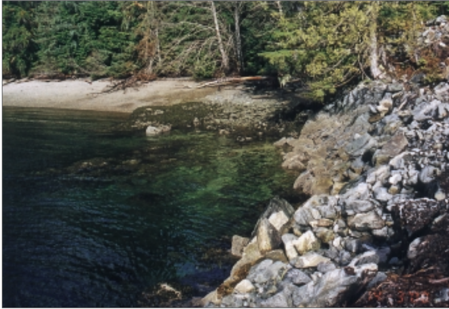
Photo 41: Verney Pass Creek dumpsite, fill on western edge placed mainly above high tidal mark (March 2000).
