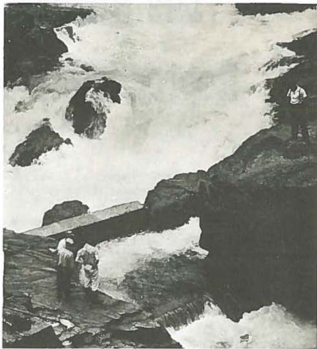
Fish ladders such as this one at Stamp Falls, B.C., help salmon move upstream.
