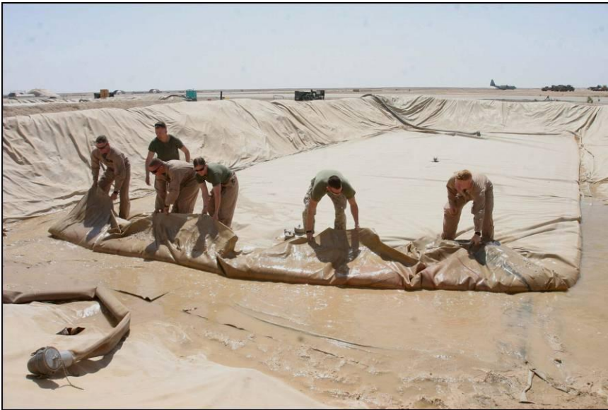
Figure 2.9. Fuel Berm with Protective Liner Installed
