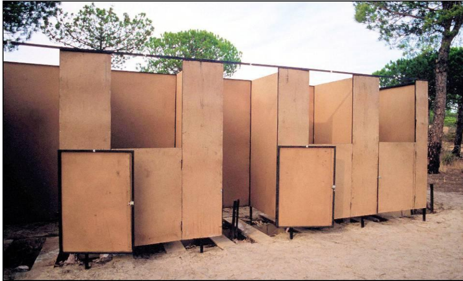
Figure 9.1. Typical Expedient Straddle-Trench Latrine with Privacy Screens
