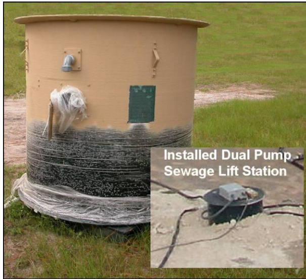
Figure 9.10. Dual-Pump Lift Station
