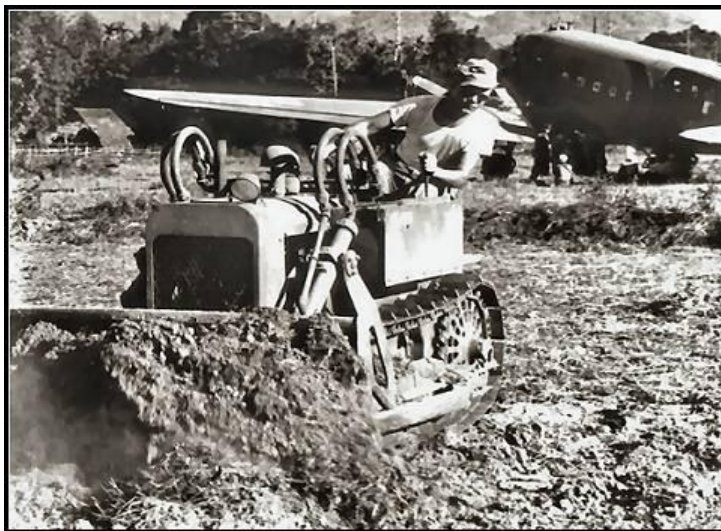
Figure 1.3. Dozer Clearing an Airfield in World War II
