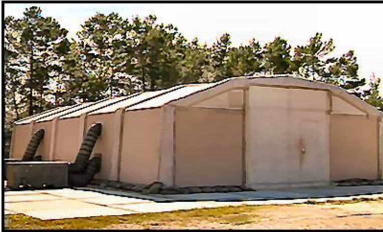
Figure 10.9. General Purpose Shelter
