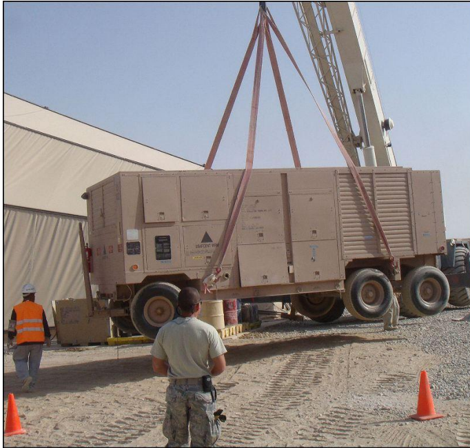
Figure 1.4. Prime Power Generators Support Sustained Operations
