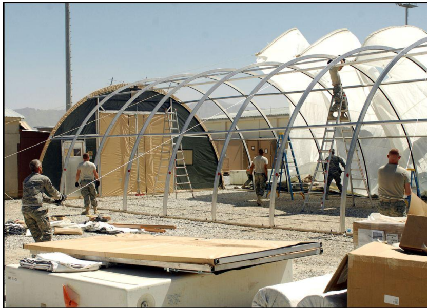
Figure 5.1. Engineer Team Assembling a Medium Shelter System
