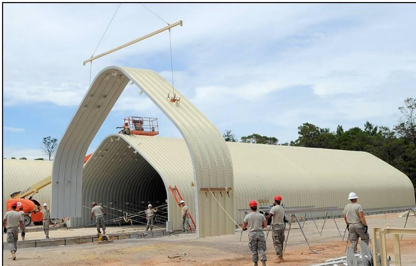
Figure 10.7. RED HORSE Crew Assembling a K-Span Building
