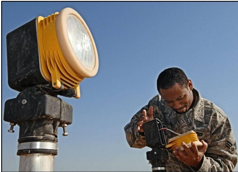
Figure 2.11. Installing Airfield Lighting - Priority 1 Task
