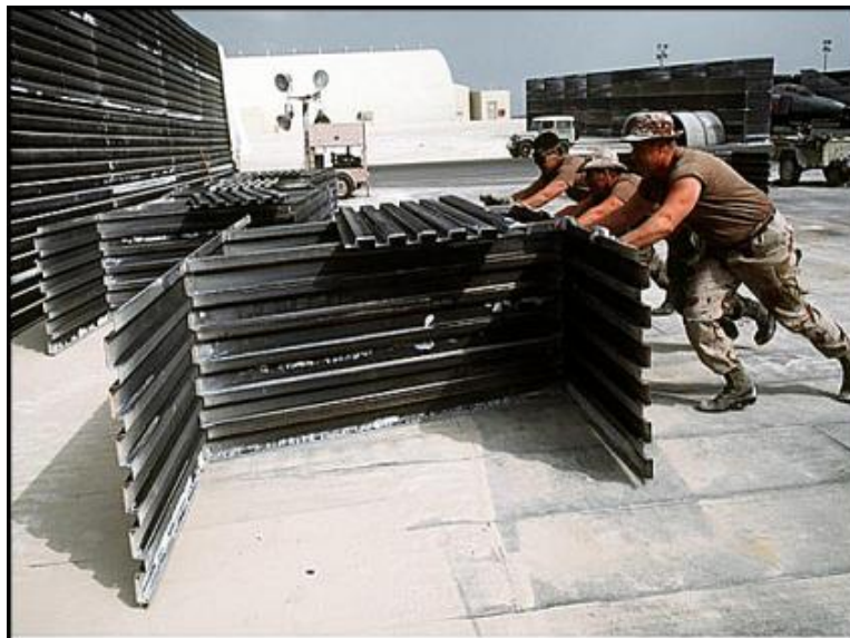
Figure 6.13. B-1 Revetment Being Assembled
