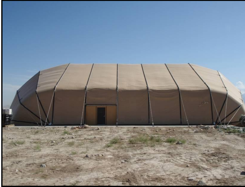
Figure 10.6. Large Area Maintenance Shelter
