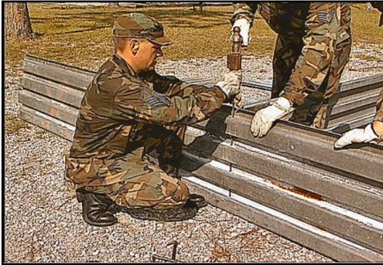
Figure 6.14. B-1 Revetment Being Pinned Together
