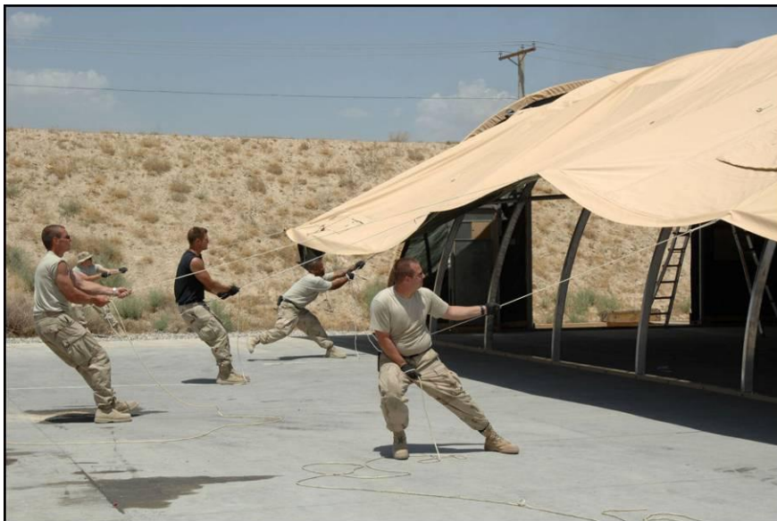
Figure 2.10. Civil Engineers Erect Medium Shelter System
