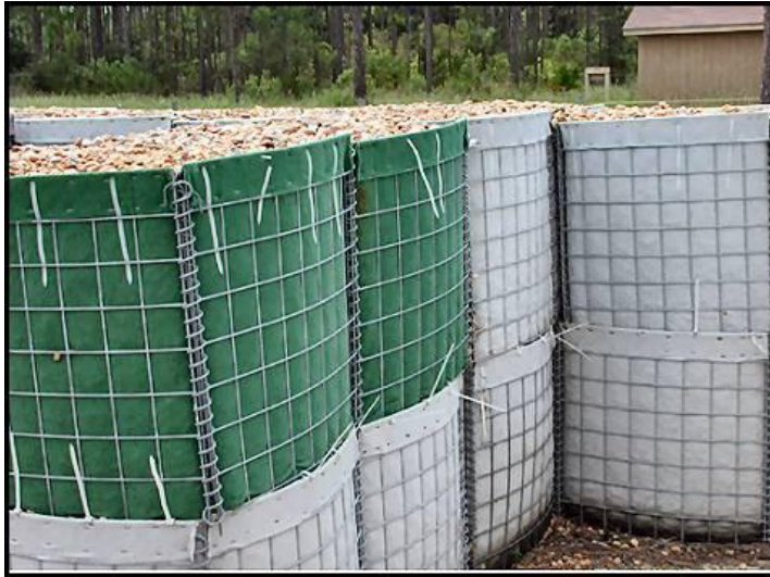
Figure 4.6. Concertainer® Revetment Material
